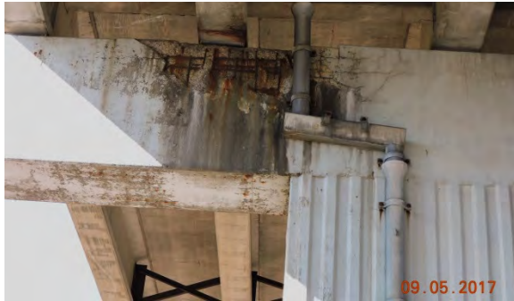
Photo 1. Cantilever pier cap cracking & deterioration. (no traffic loads can be supported by cantilevers)
