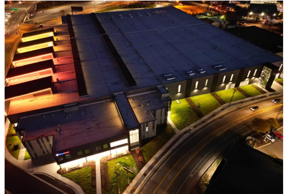
View of North Loop Garage exterior
