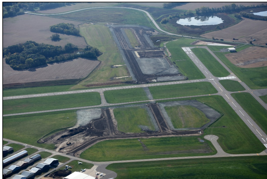
Current 2021 photo showing the Runway 14-32 Relocation/Extension and Associated Improvements construction site.
