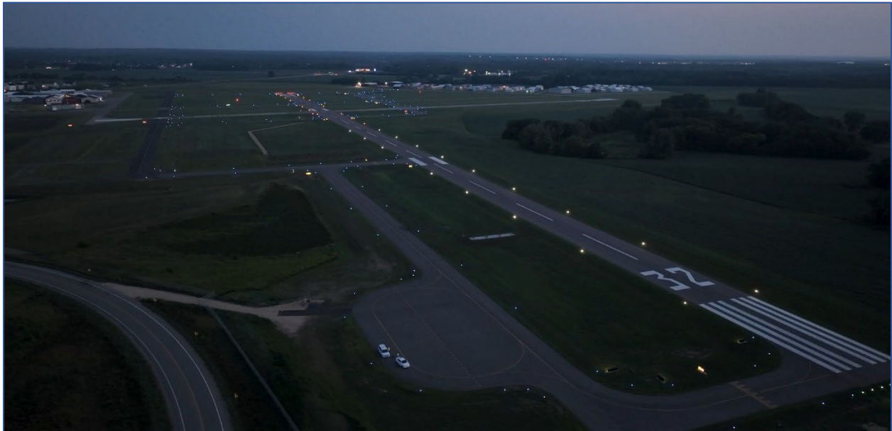
An early evening view of the realigned Runway 14-32
