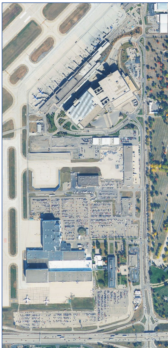
MSP Terminal 2 and Delta Air Lines Office Complex
