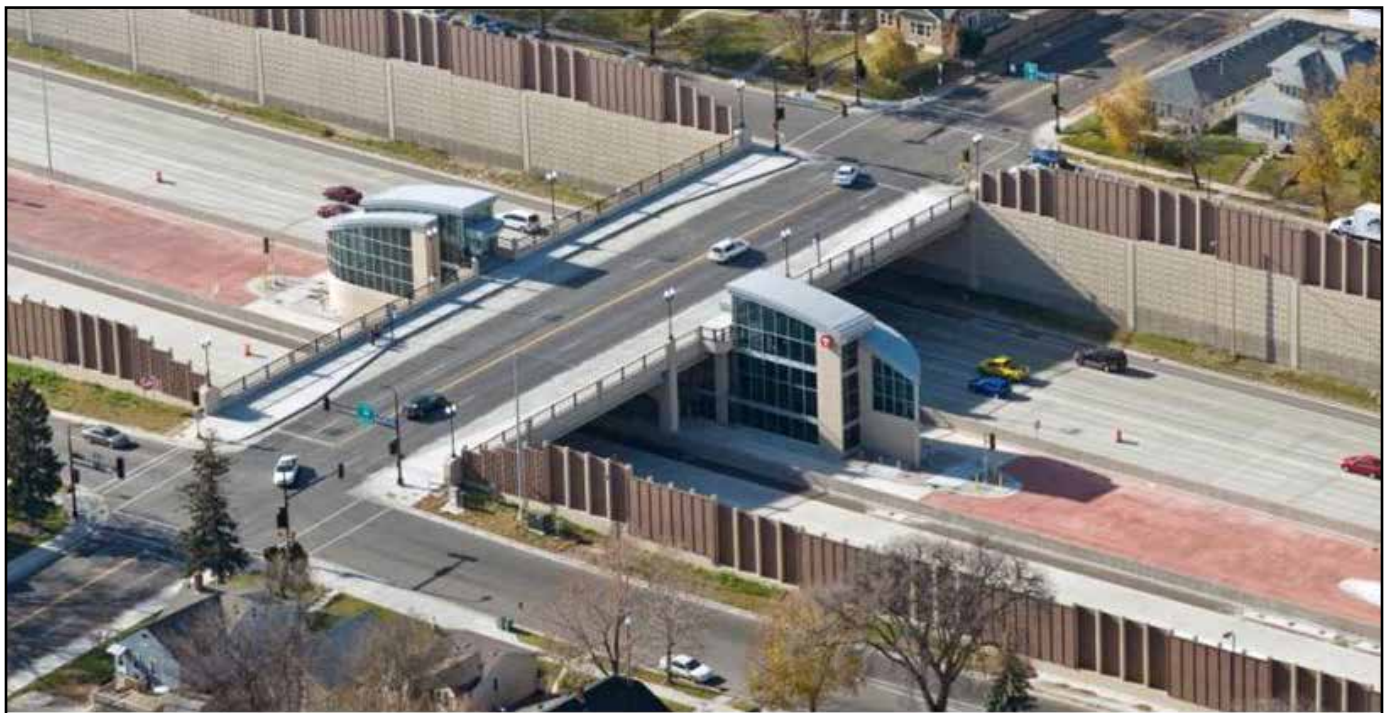
Figure 10. Aerial View of 46th Street Station
