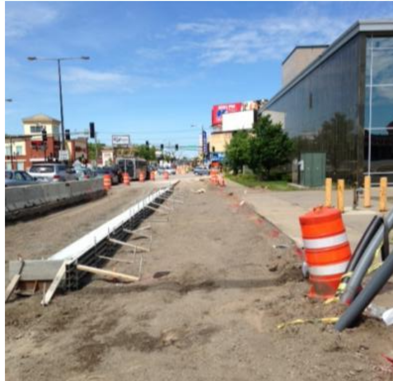
Snelling & University – Northbound Looking north (June 1)
