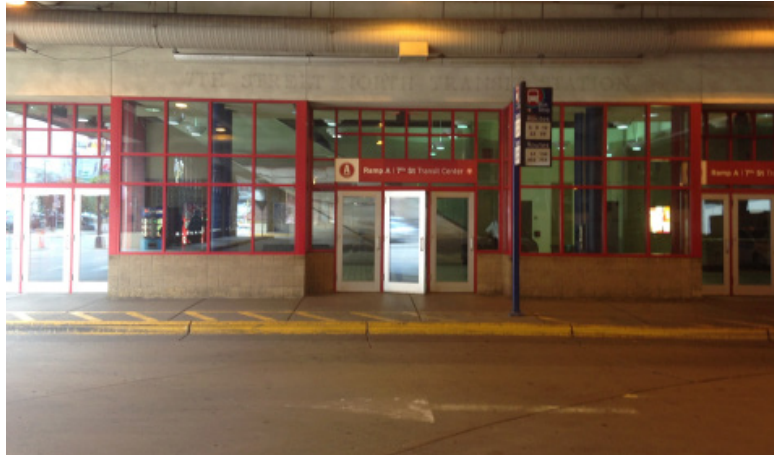
Figure 1: Existing Ramp A/7th Street Transit Center
