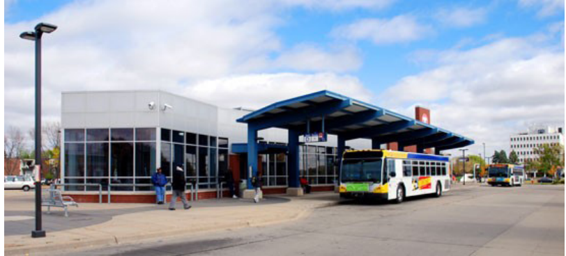
Figure 1: Brooklyn Center Transit Center
