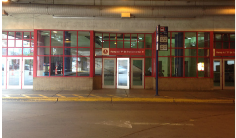
Figure 1: Existing Ramp A/7th Street Transit Center
