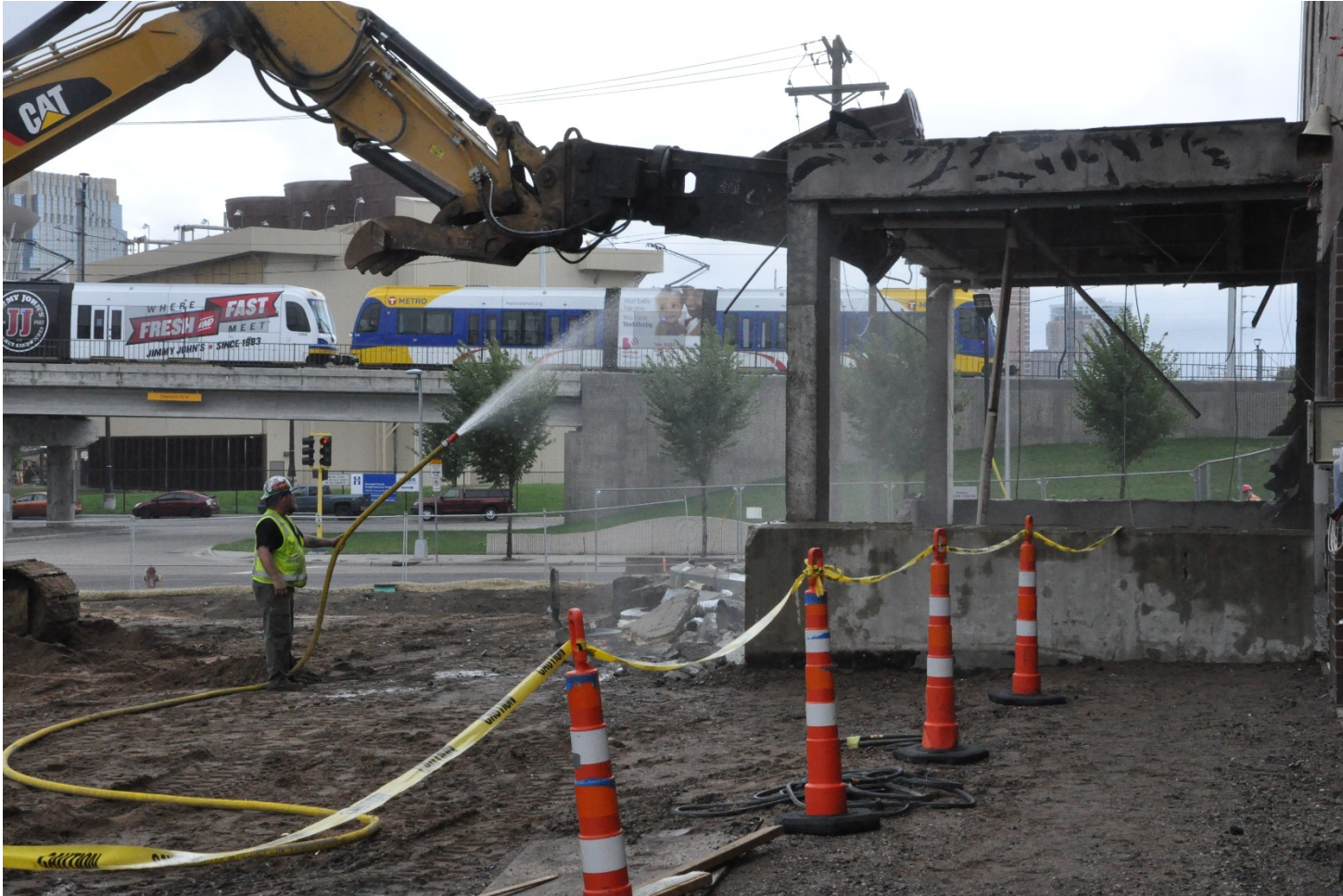
Partial Building Demolition
