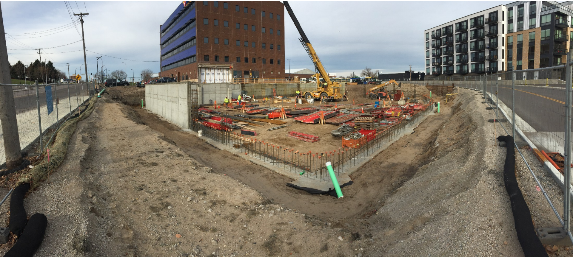
Foundation Wall Framing
