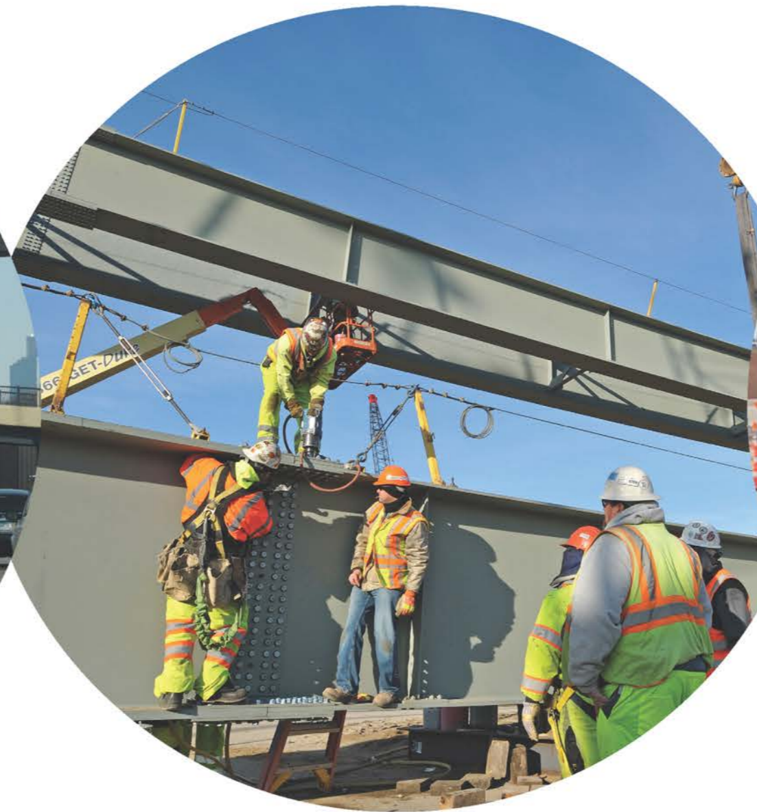
Replacing or preserving aging roads for safety and reliability
