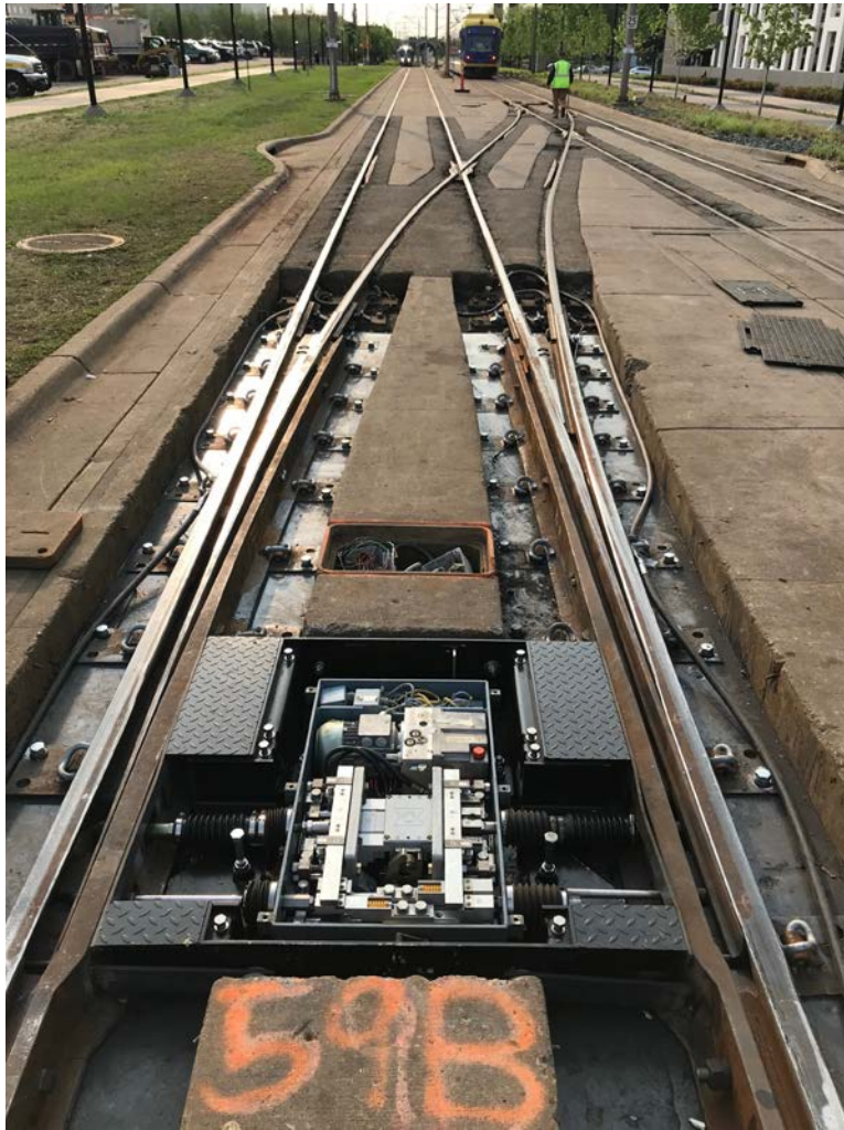
Existing embedded track at 28 th Ave Interlocking.
