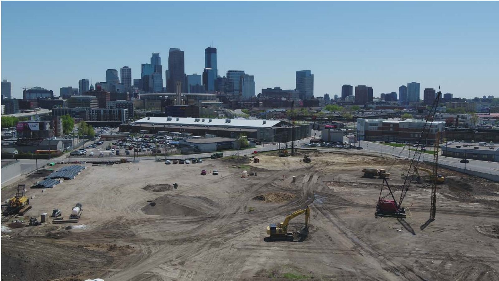
Week 2 of construction
