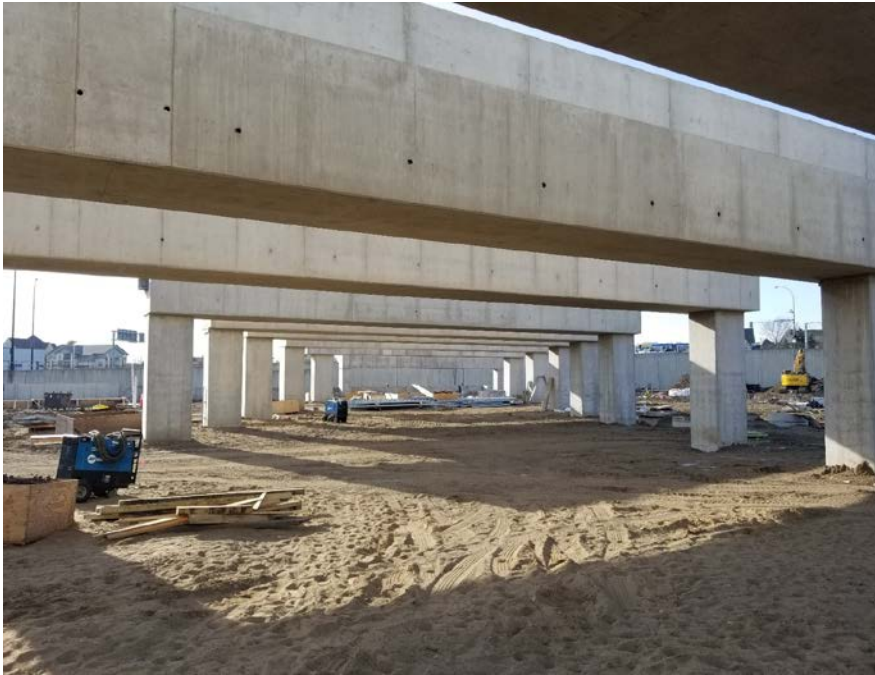
Transfer girders over Bassett Creek stormwater tunnel
