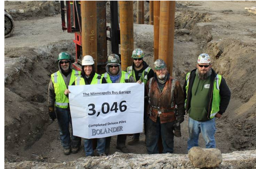
Pile driving construction crew
