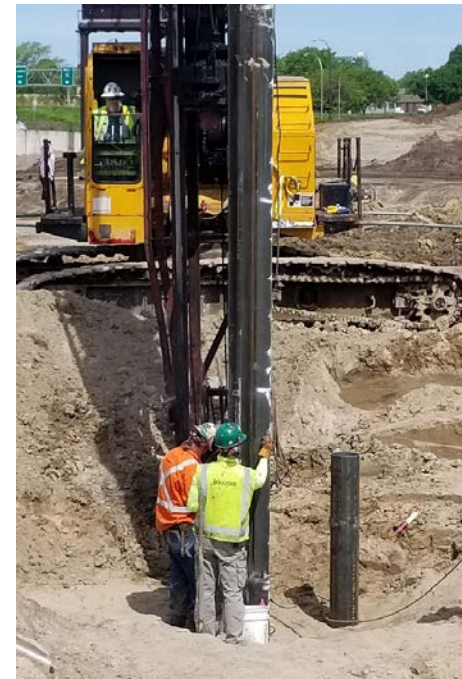
DBE pile driving observation
