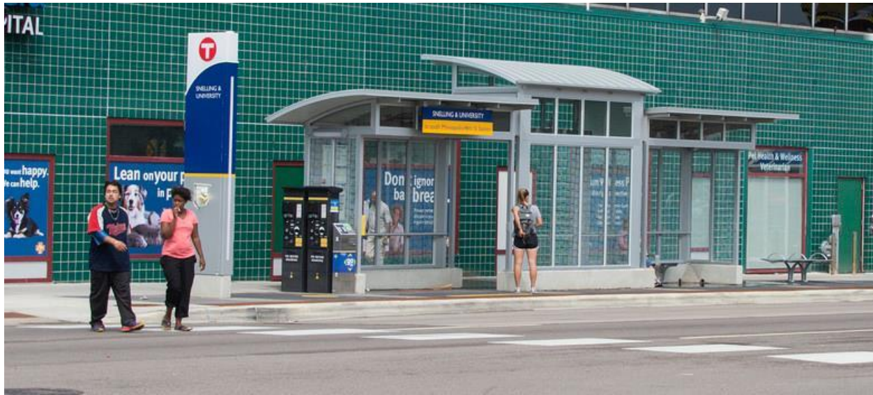
Figure 21: Large shelter on the A Line, Snelling & University Station
