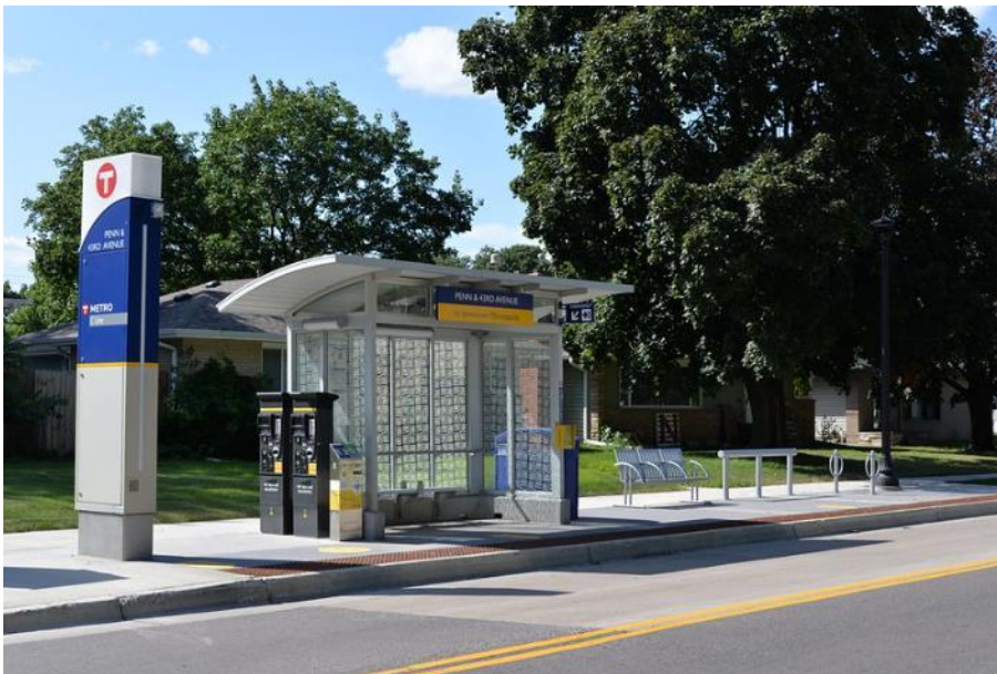
Figure 8: Arterial BRT shelter
