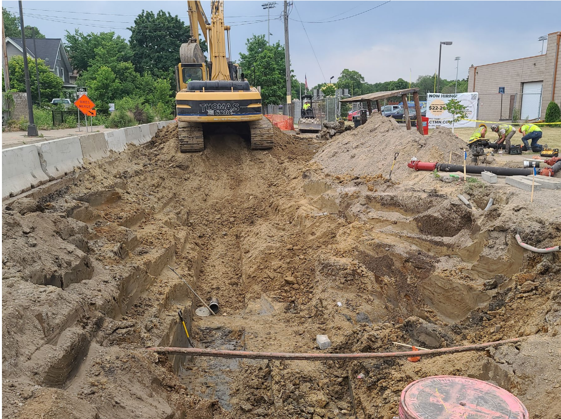
Removals & underground utility work at Fremont & Broadway
