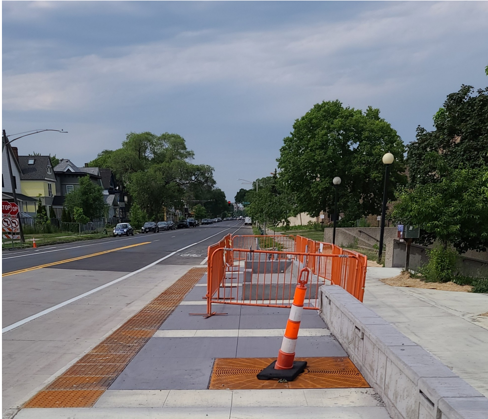
Substantially complete platform at Chicago & 34th Street
