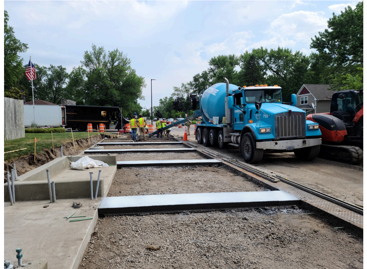
Station platform concrete pour at Portland & 73rd Street
