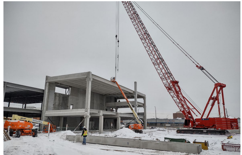
Four pictures of precast concrete being placed for new garage construction
