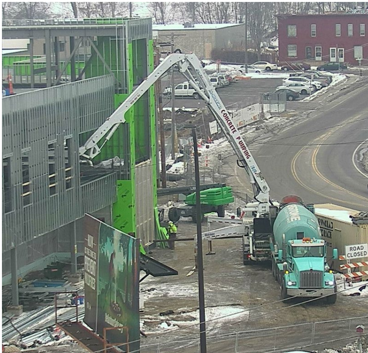
Concrete Pumping – DBE
