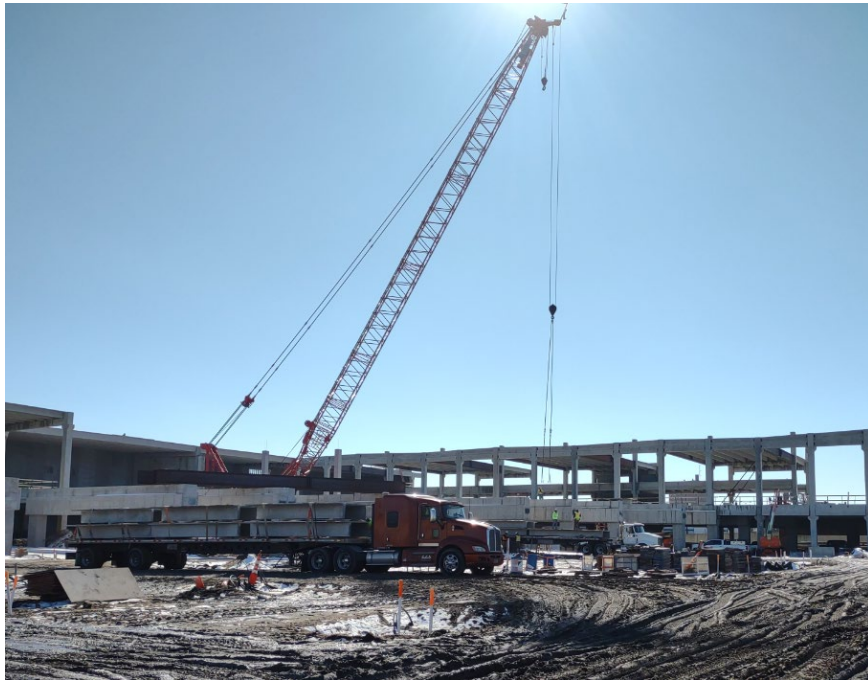
Crane picking precast concrete, building in background
