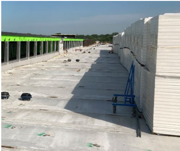
Roof construction, roof insulation
