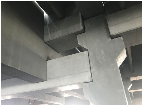
3 pictures of bus lifts structural framing
