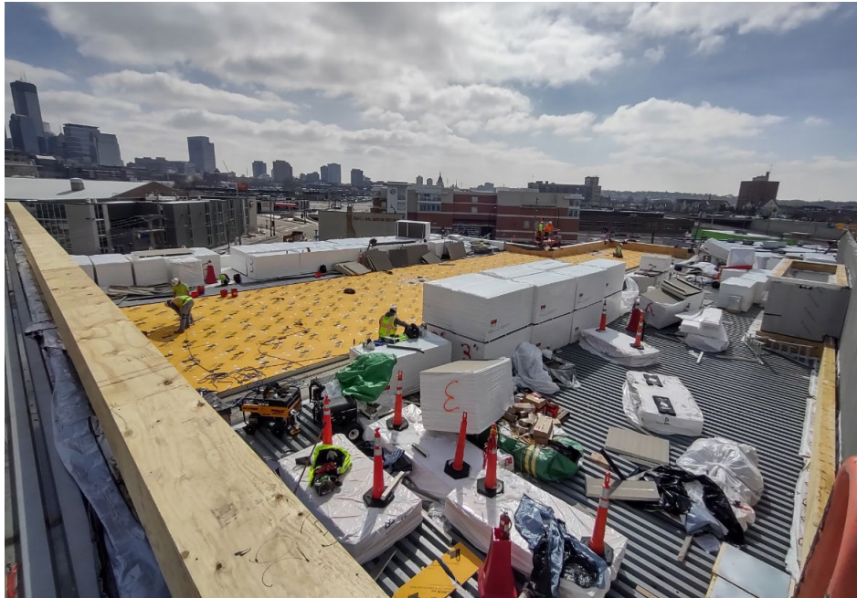
Roof materials and crew installing
