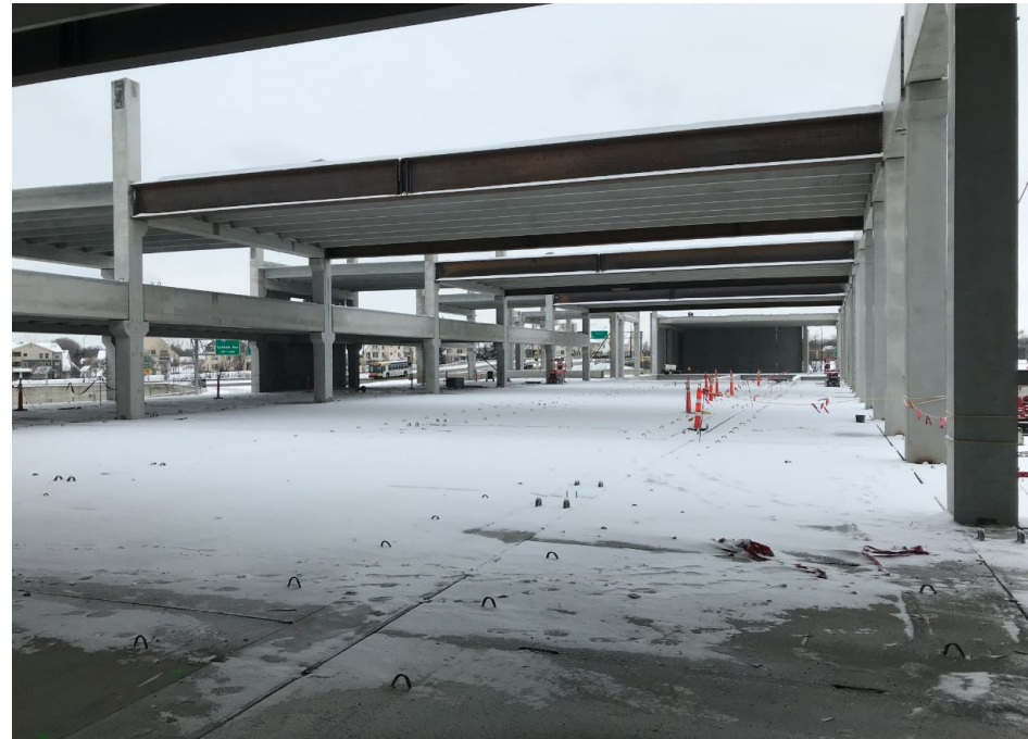
Inside picture of building with structural framing
