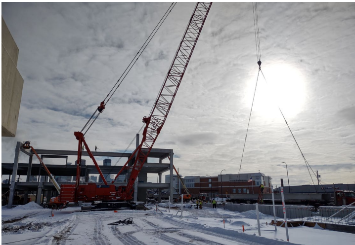
Four pictures of precast concrete being placed for new garage construction
