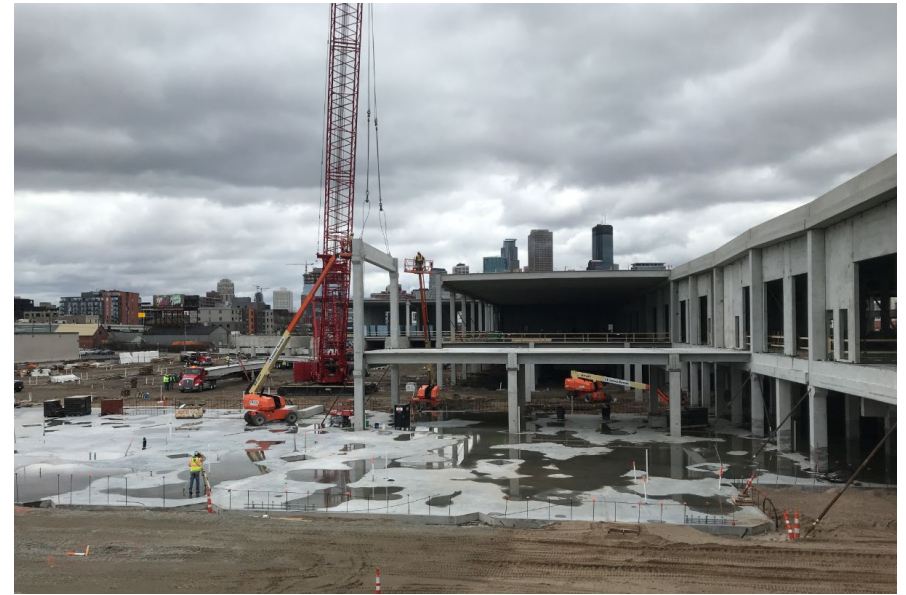
Exterior pictures of bus garage showing façade/windows going in and pre-cast beam being placed by crane.
