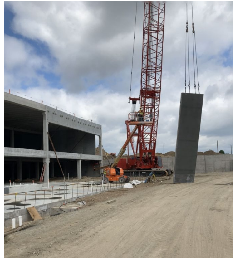
Precast panel being lifted by crane
