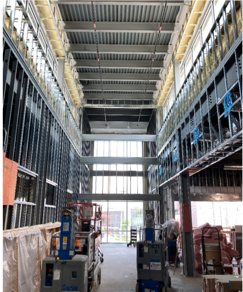
Interior building construction
