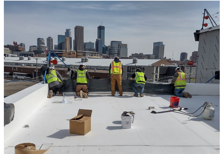
Roofing installation - DBE
