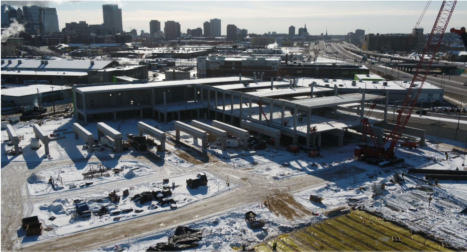
January 2021 Site picture of bus garage structural framing
