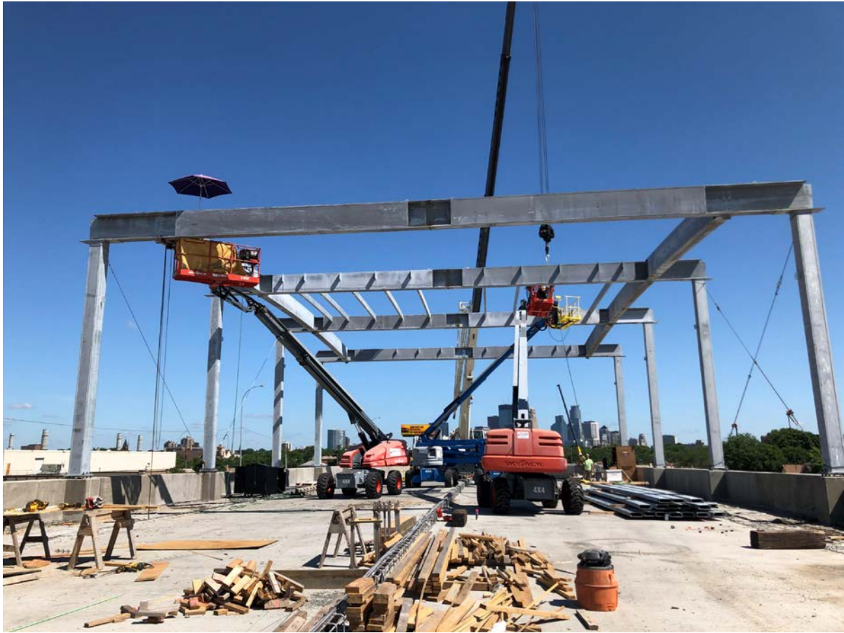
Bald Eagle Erectors Installing Lake Street Canopy, Summer 2020
