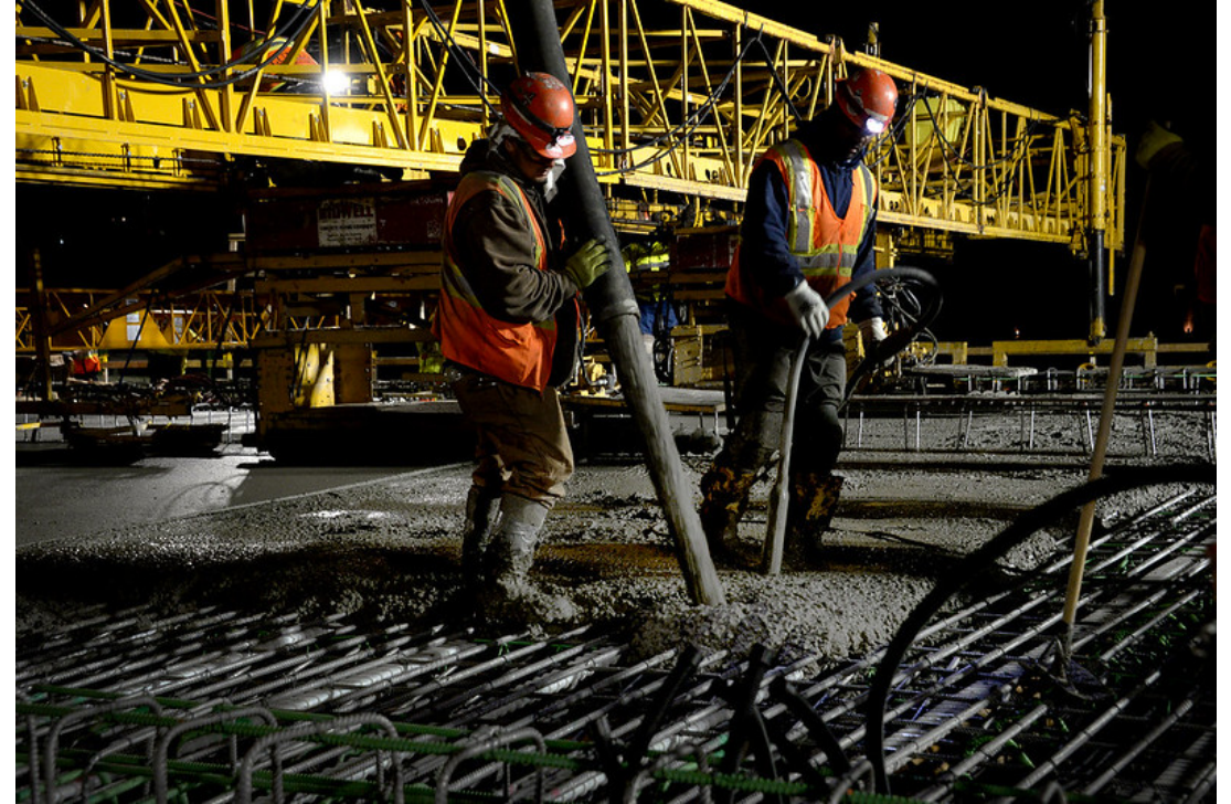
Pouring of the Transit Bridge, Fall 2019
