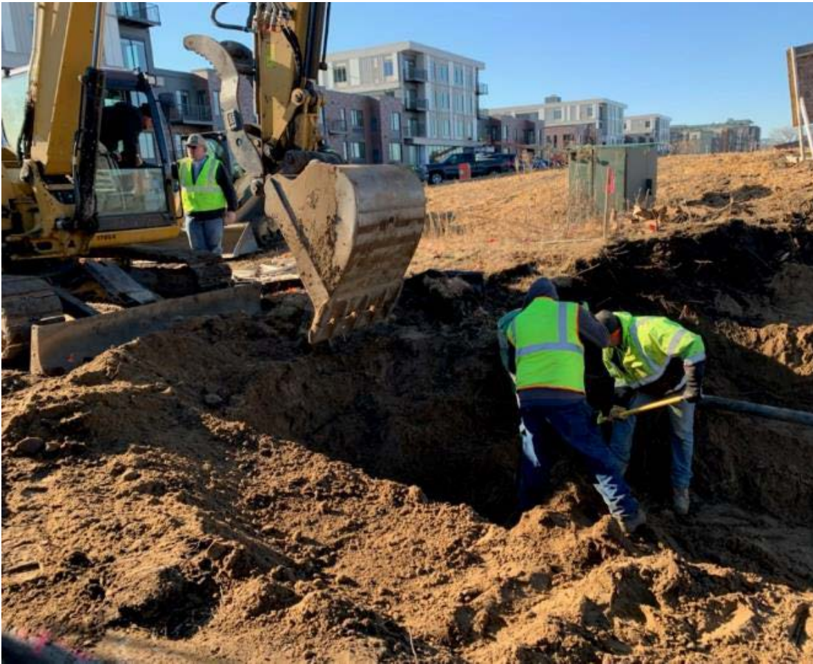
Southbound Knox and American Station utility installation, Fall 2020
