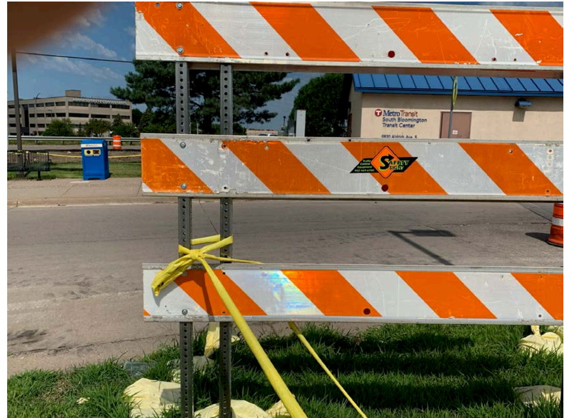
Safety Signs installing signage, Summer 2020
