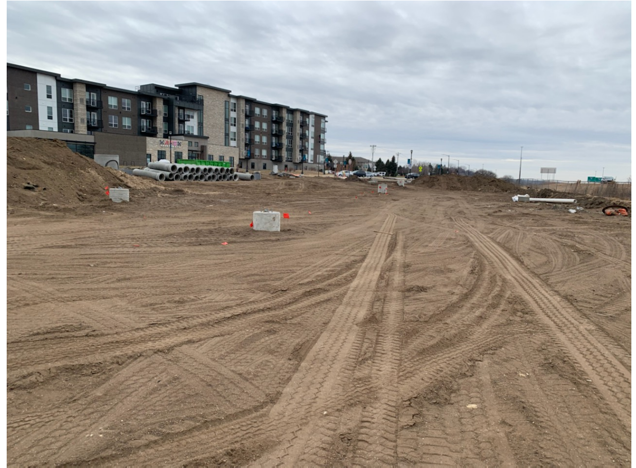
Burnsville Heart of the City Construction, Fall 2020
