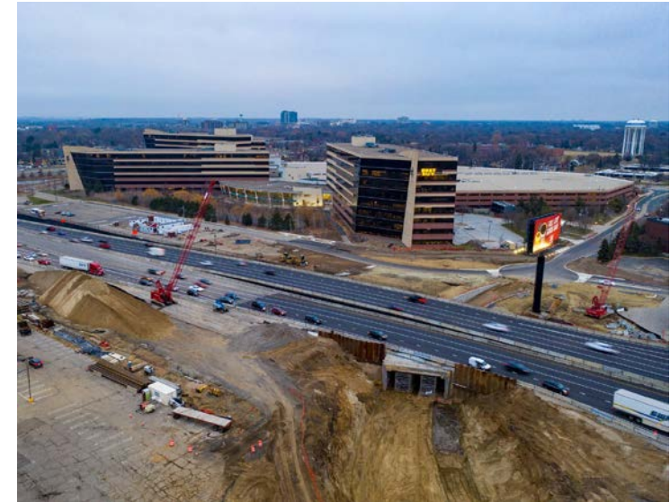
North half tunnel complete, Fall 2020
