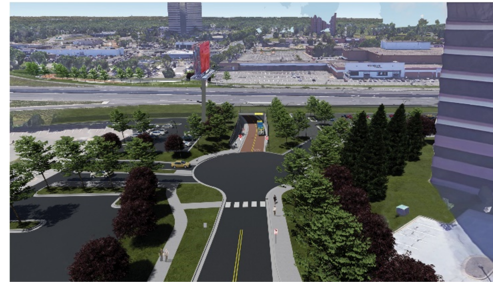
Final Condition Looking south
