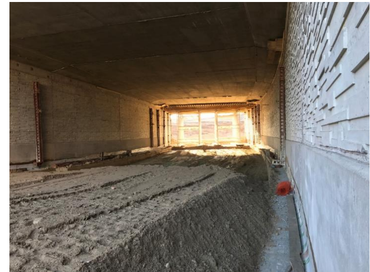
North half tunnel interior, Fall 2020
