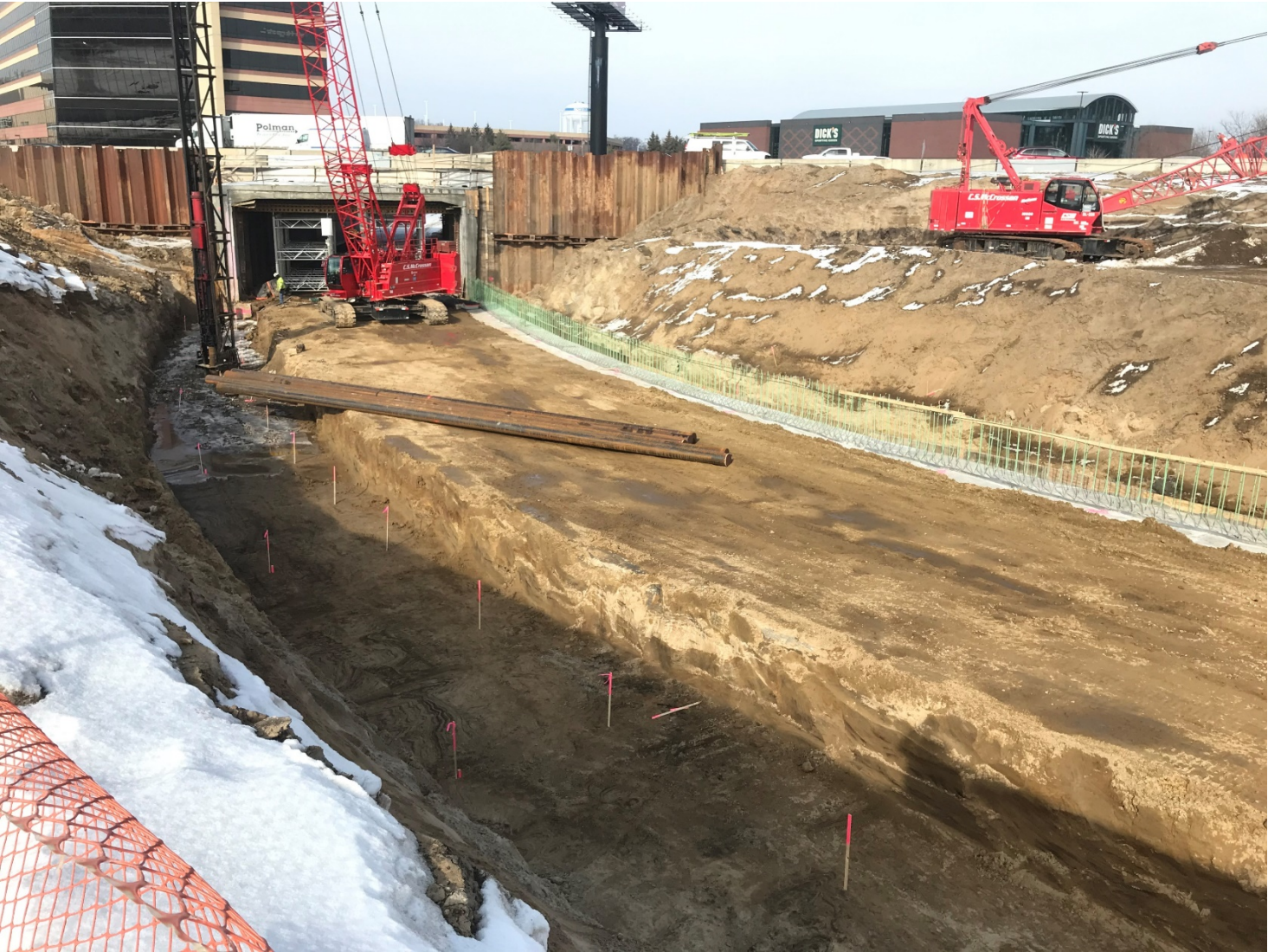
South half tunnel piling west wall , Winter 2021
