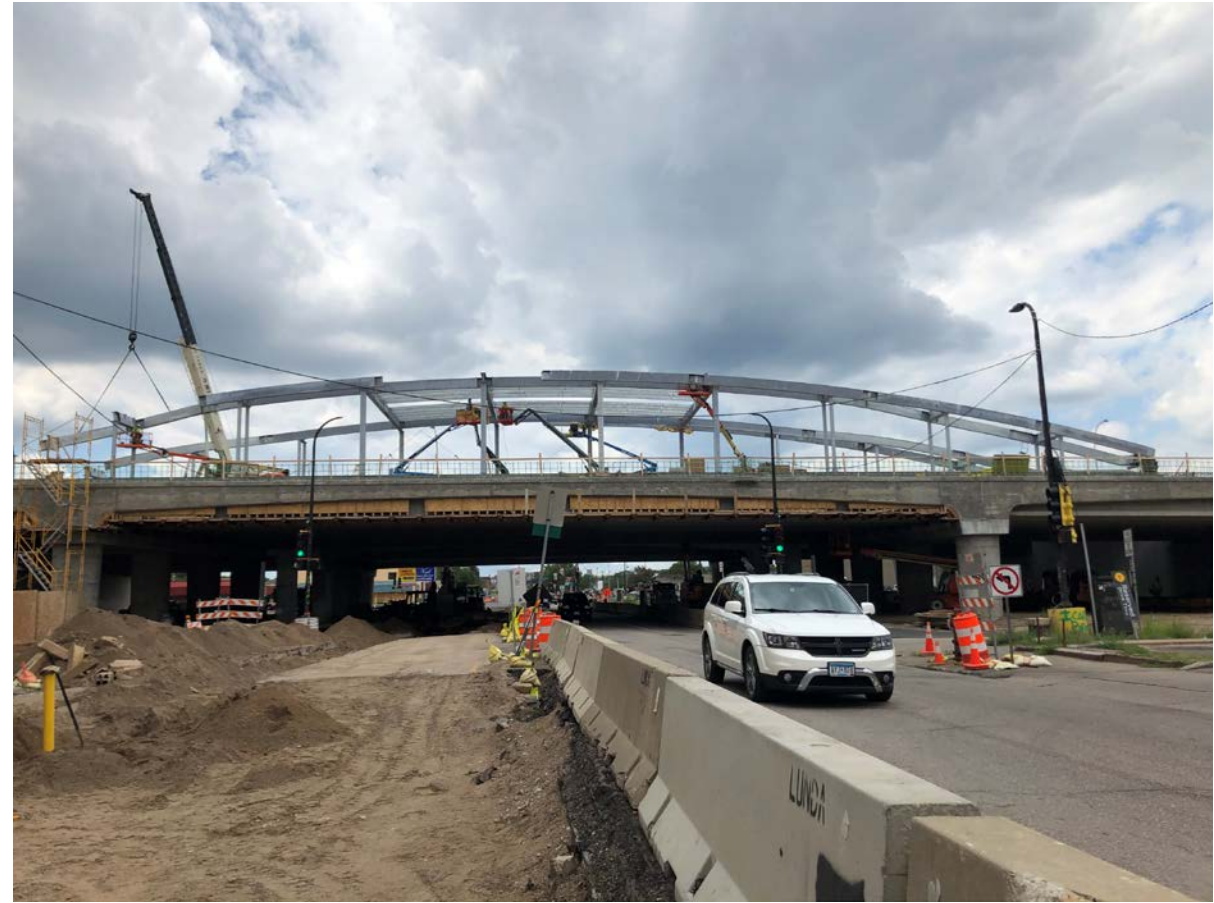
Bald Eagle Erectors Installing Lake Street Canopy, Fall 2020
