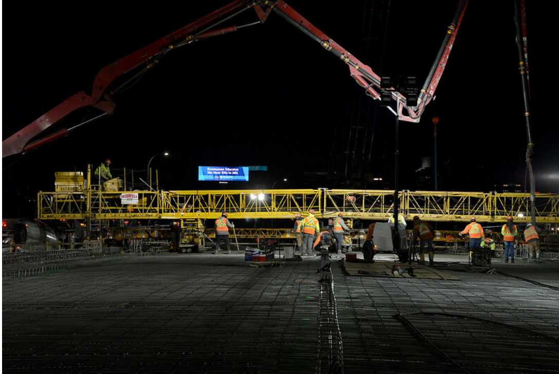
Pouring of the Transit Bridge, Fall 2019
