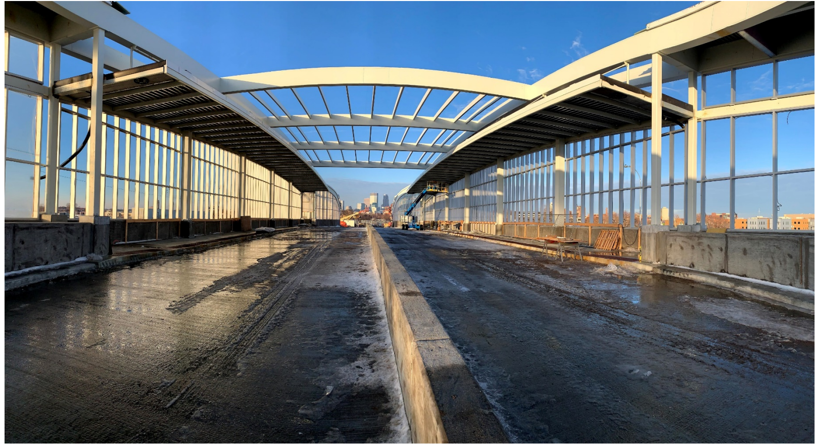
Transit Bridge, Winter 2021
