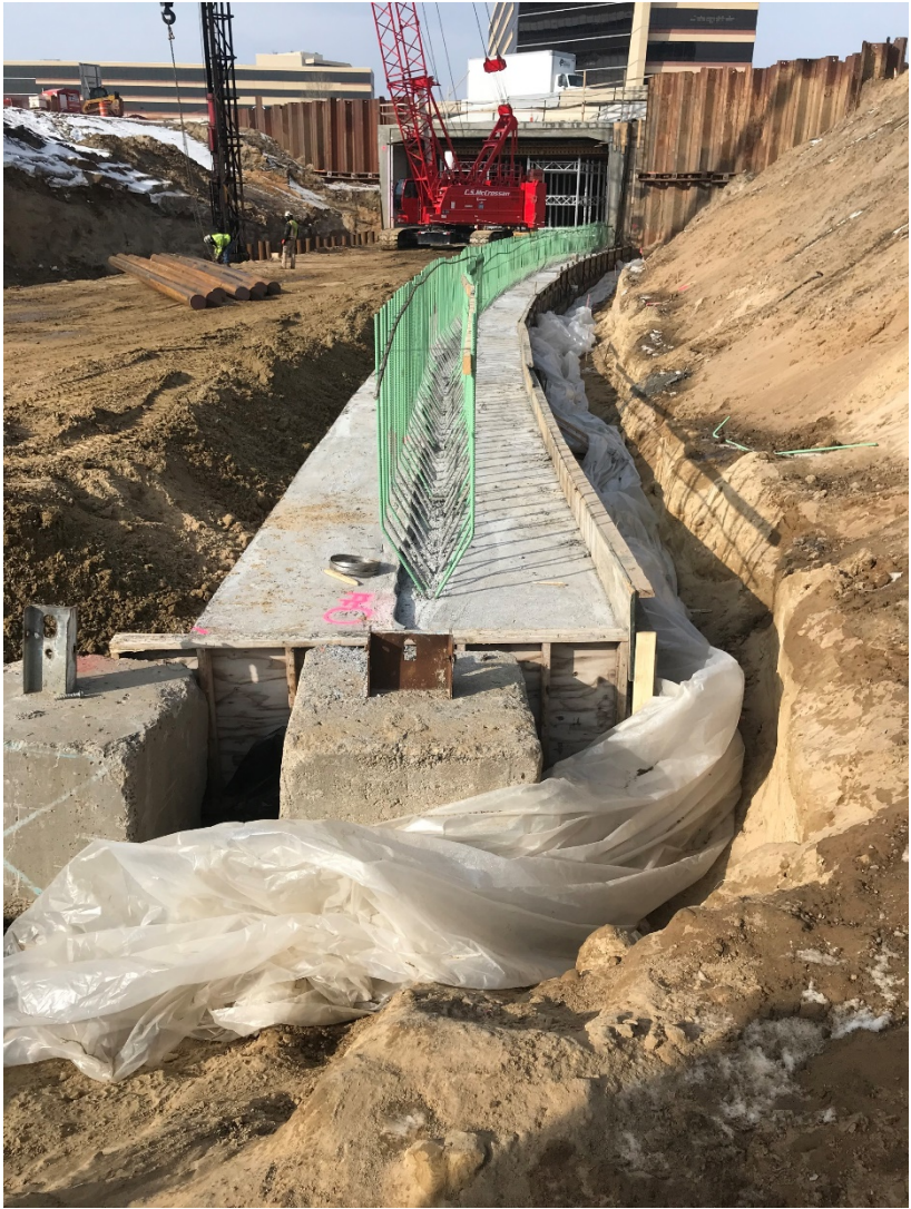
South half tunnel east walls foundation, Winter 2021
