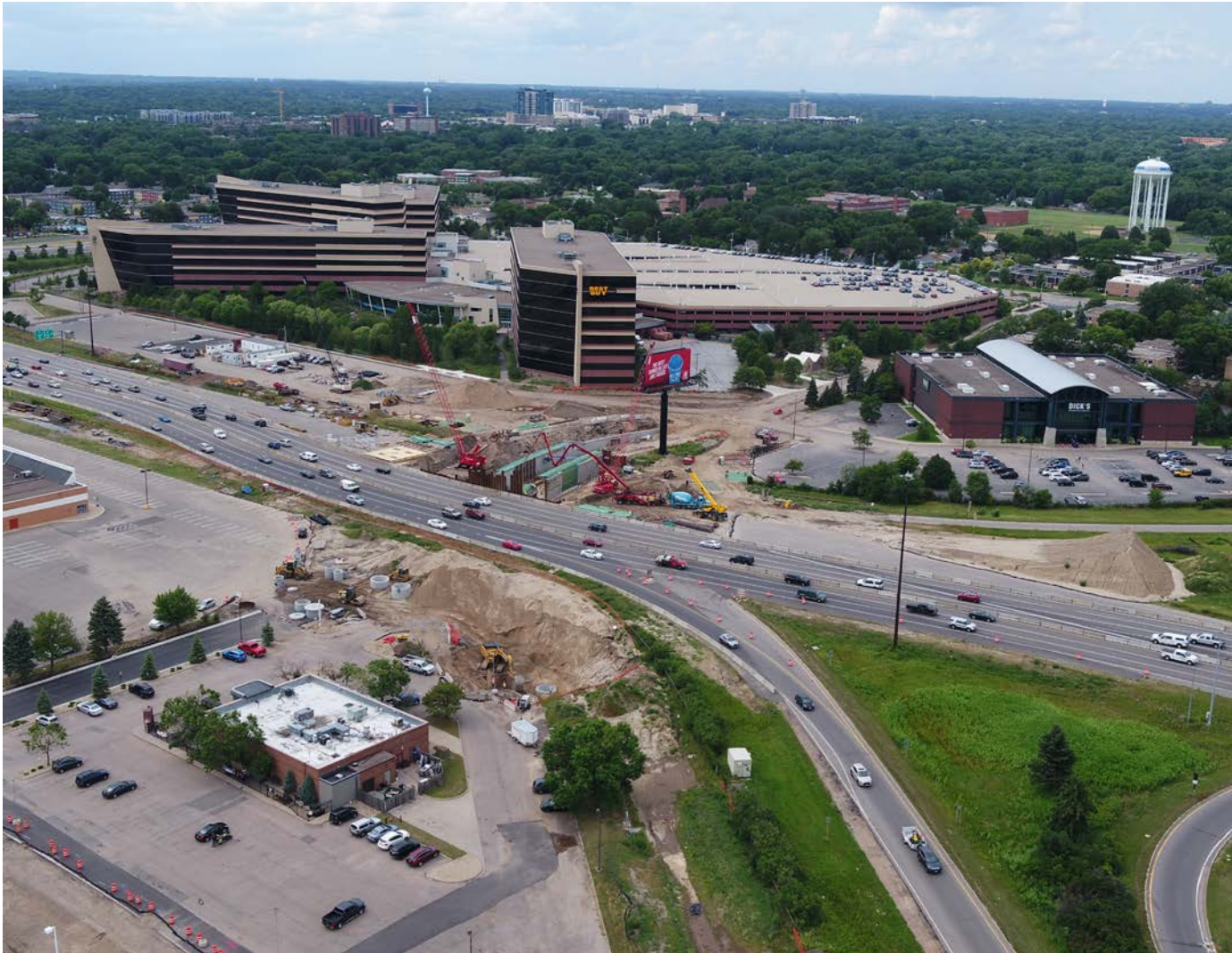
North half tunnel construction, Summer 2020
