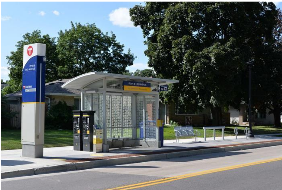
Figure 8: Arterial BRT shelter
