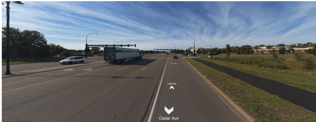
Figure 3: Southbound CSAH 23 (Cedar Avenue) at CSAH 46 (160th Street West)
