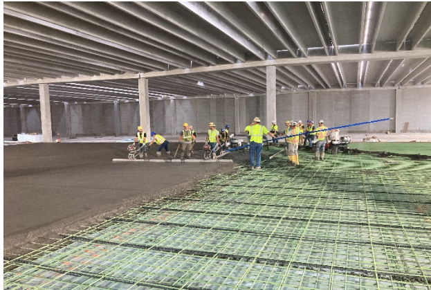
Concrete Slab Installation
