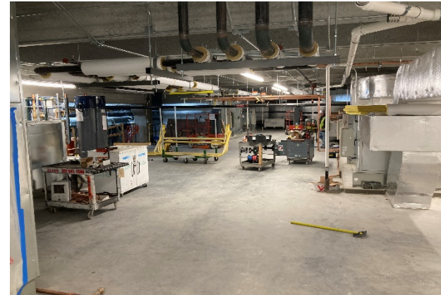
Construction within Mechanical Mezzanine
