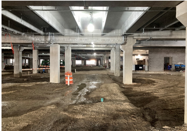
Street Level Parking Area
