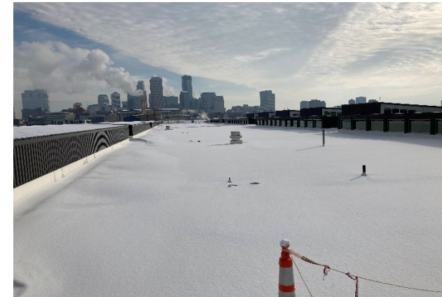
Snow on Completed Section of Roof
