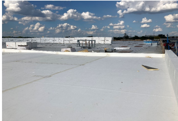
Waterproofing and Insulation Installation
