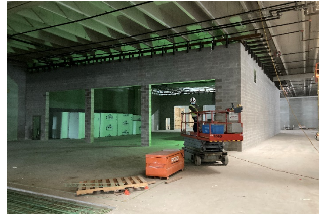
Interior Wall Installation Complete
