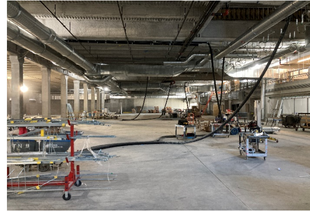
Construction within Mechanical Mezzanine
