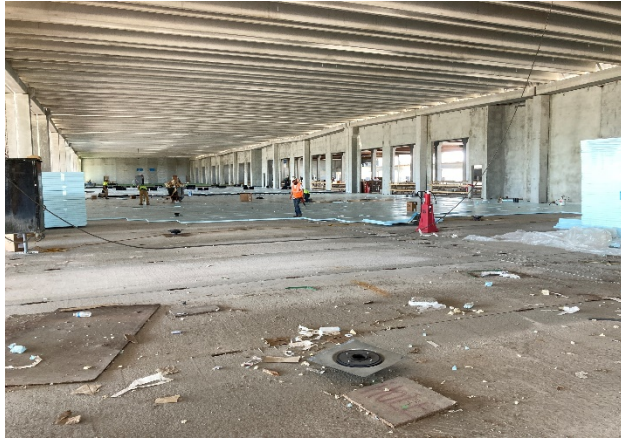
Insulation of Main Level
