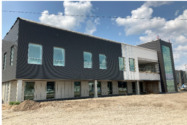
Exterior Wall Finishing
