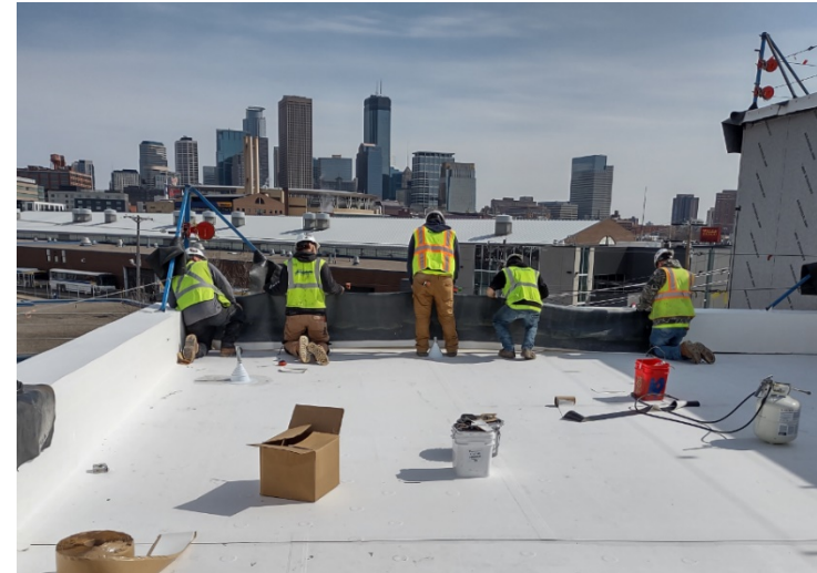
Roofing installation - DBE
