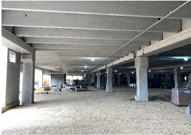
Street Level Parking Area
