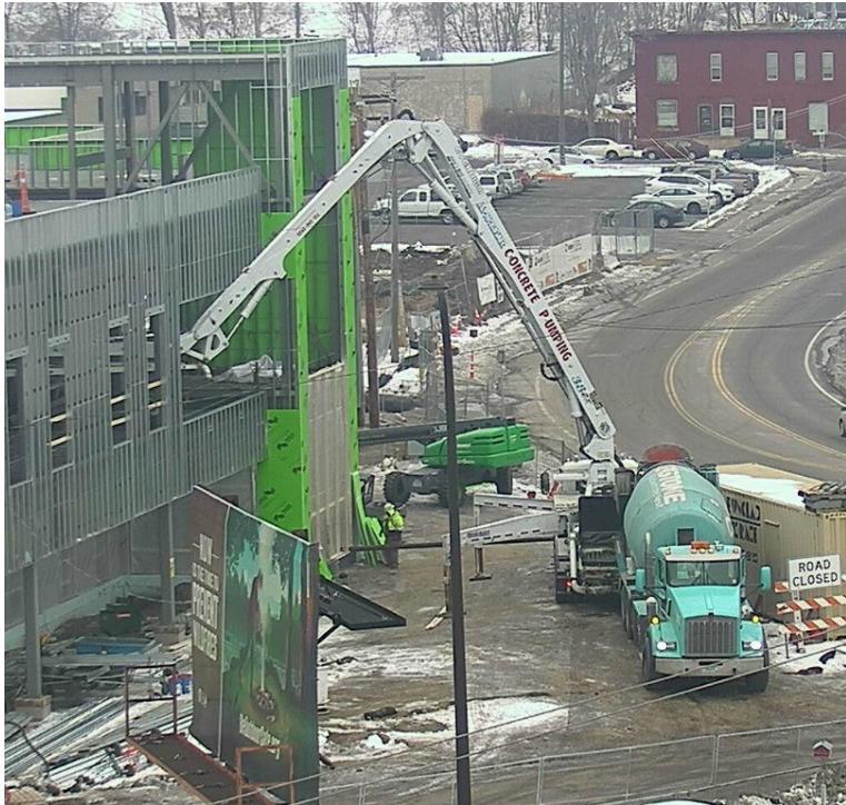
Concrete Pumping – DBE
