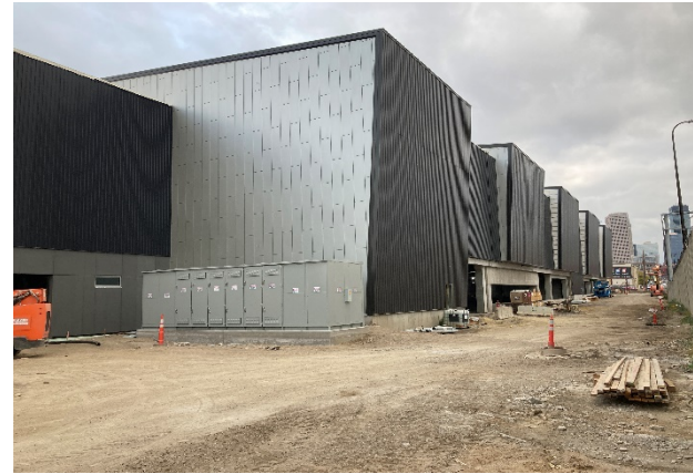
Finished Exterior of the South Wall
