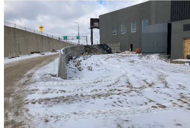
Completed Retaining Wall
