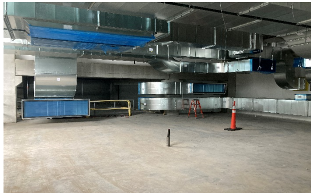
Ductwork Installation
