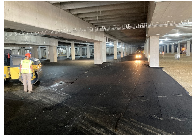
Parking Area Pavement Installation
