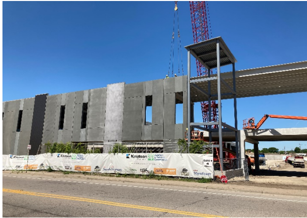
Pre-cast Wall Installation
