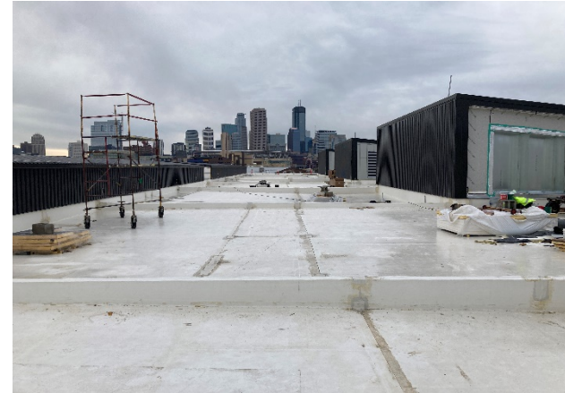
Wrapping up the Installation of a Roof Section
