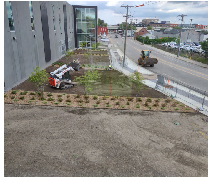
Completed Retaining Wall
