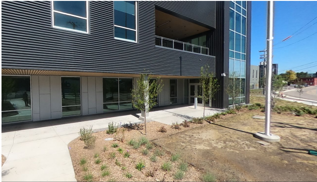
Exterior Wall Finishing
