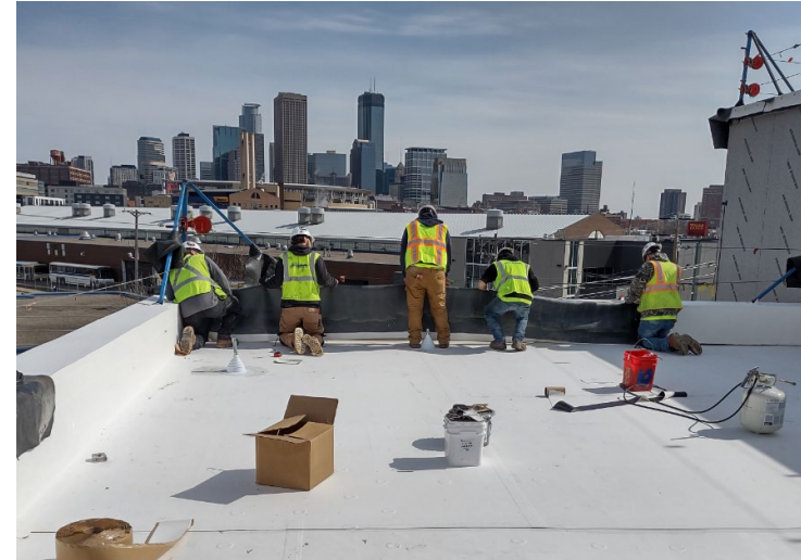
Roofing installation - DBE
