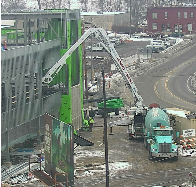
Concrete Pumping – DBE
