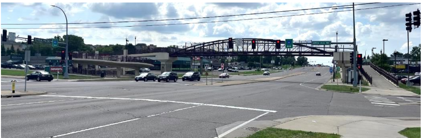
View south down Central Avenue at pedestrian bridge and proposed platform locations (Source: Metro Transit)
