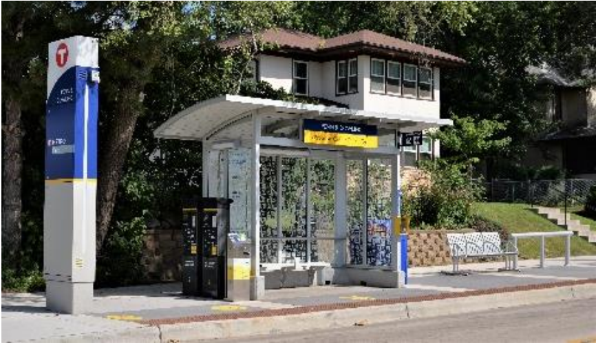
Example of a small arterial BRT shelter (Source: Metro Transit)
