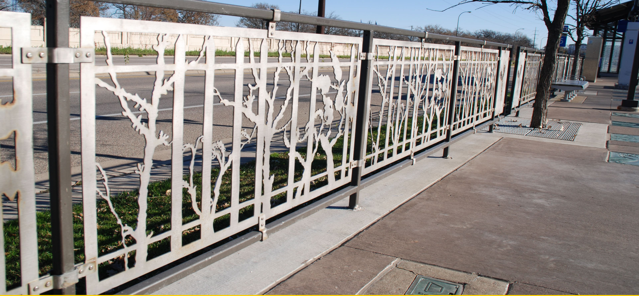
Stainless Steel Fence Repair – 50 th Street Station
