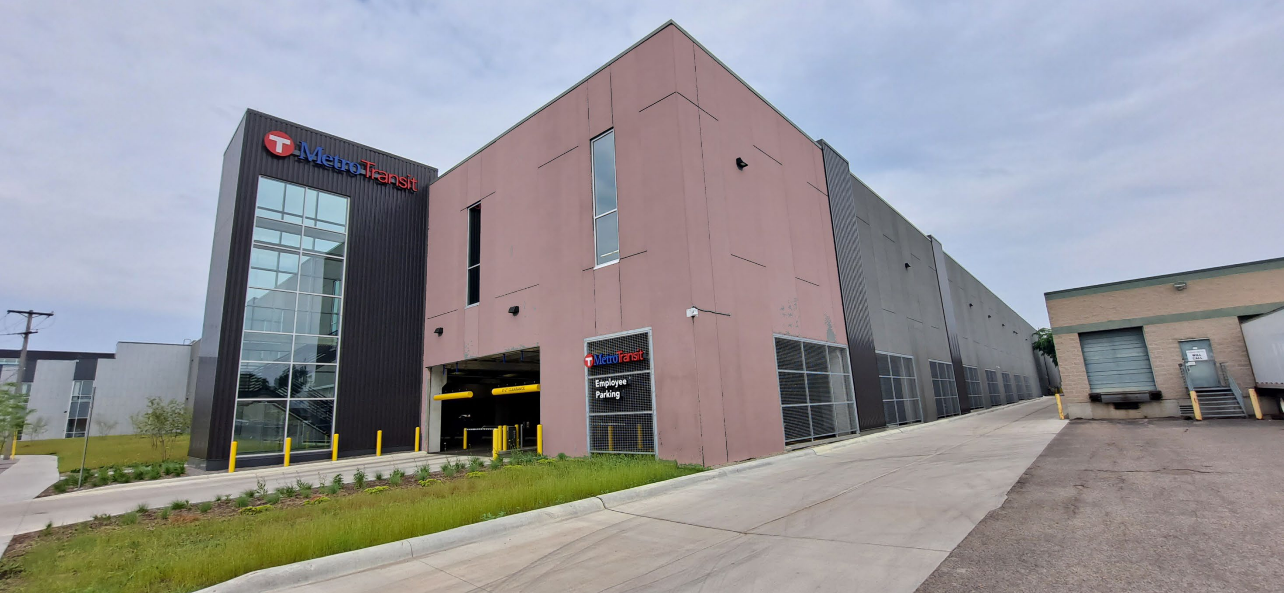
2024 North Loop Garage
