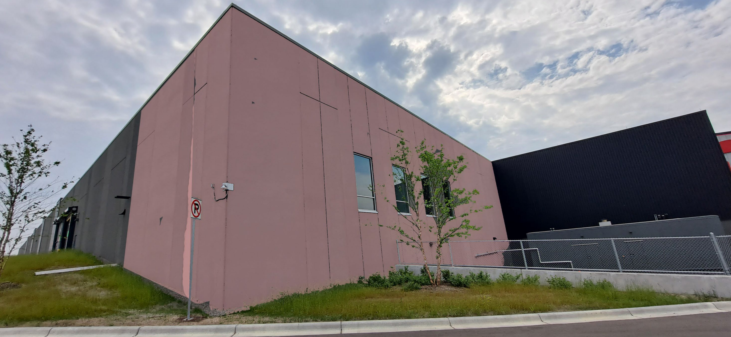
2024 North Loop Garage
