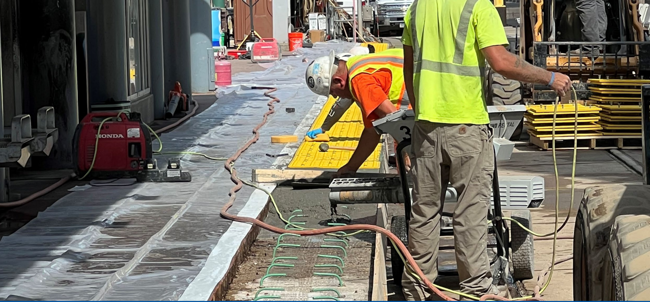
Hennepin Ave/Warehouse Station Work – Summer 2023
