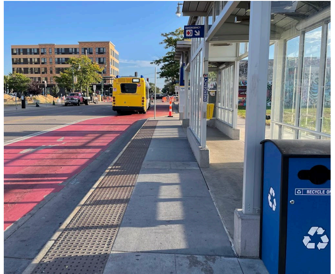
Southbound D Line station with amenities and bus on Chicago Ave at Transit Center 4
