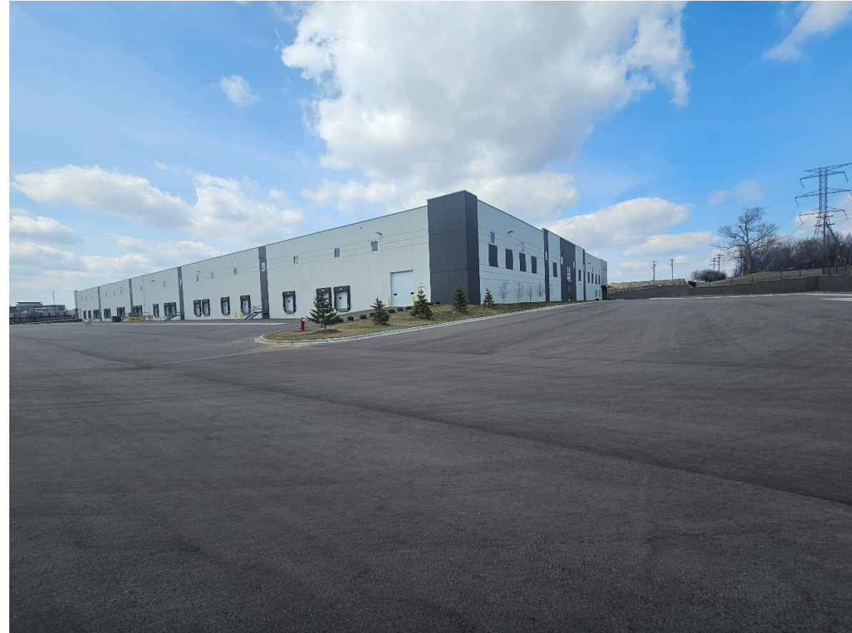
Southeast exterior elevation of building
