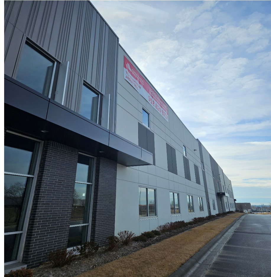
West exterior elevation of building
