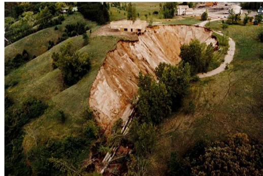
Figure 2: Interceptor failure - Minnesota River
