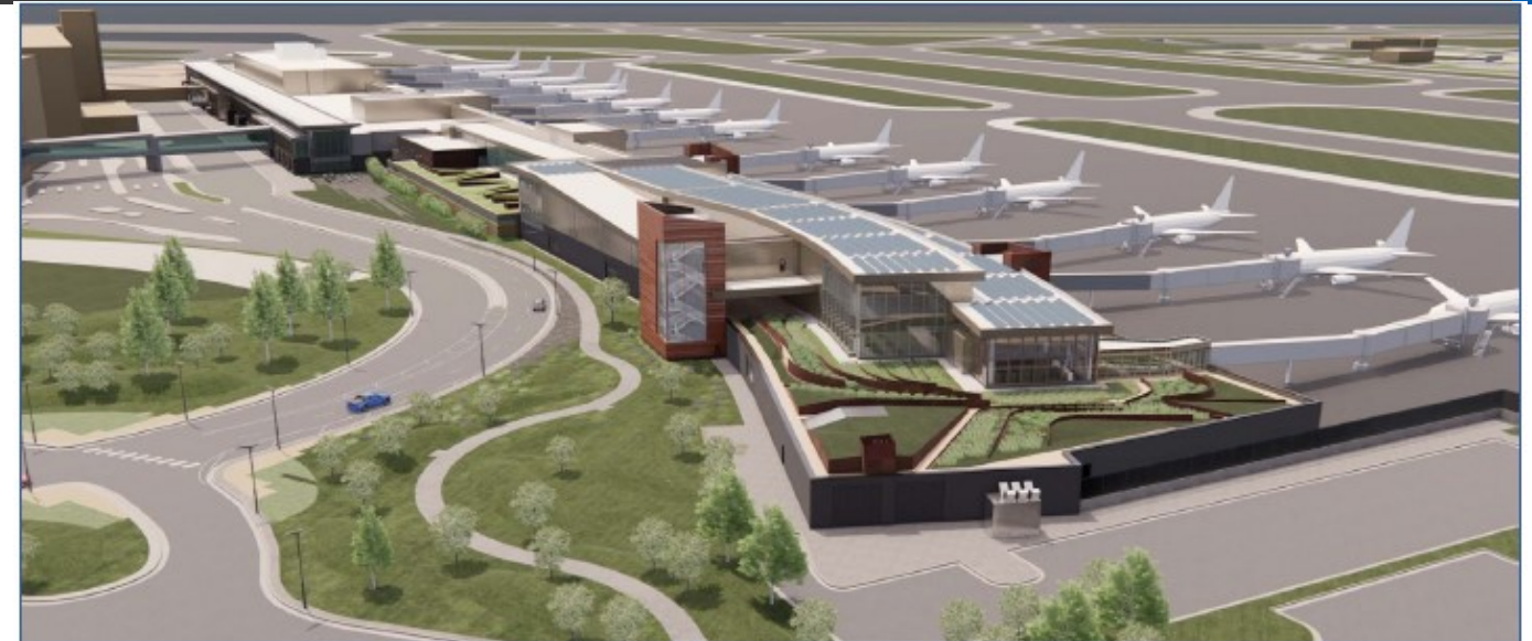
*Rendering of Terminal 2 expansion set to begin construction in 2024
