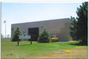
FIGURE 6-2 OSSEO PUBLIC WORKS BUILDING
