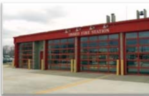
FIGURE 6-5 OSSEO FIRE STATION
