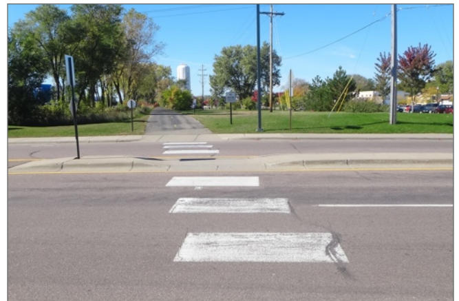
A marked crosswalk and small pedestrian refuge help indicate the importance of the Minnesota River Bluffs Trail crossing at this intersection with 5th Avenue South.
