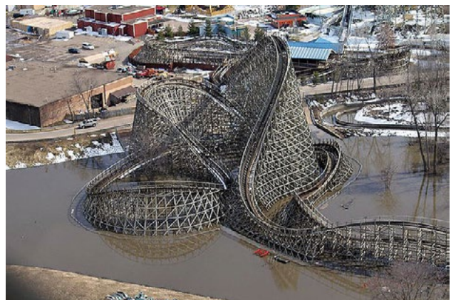
Renegade rollercoaster at Valley Fair submerged in floodwater, 2011 Source: MPR News
