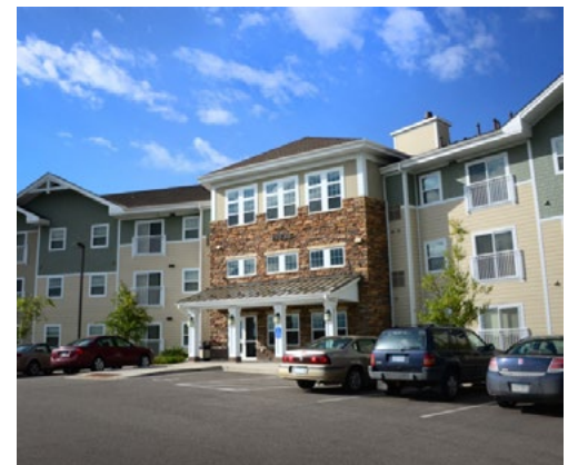
Headwaters Workforce Housing- The new Housing Chapter adopted stronger policies and strategies to create more affordable housing in the community.
