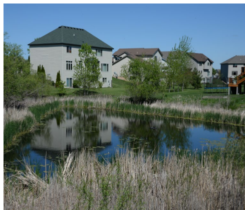
A new system was installed in the Beaver Ponds Park to pump stormwater out of nearby ponds to irrigate the park.
