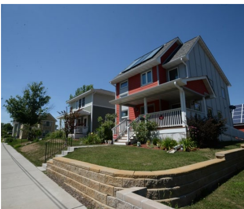
The red house to the right contains solar panels, supporting the community's efforts in becoming more sustainable.
