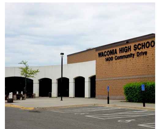
The existing Waconia High School will become Clearwater Middle School once construction of the new Waconia High School is completed.
