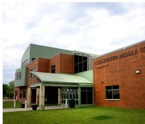
Clearwater Middle School is currently being reconfigured into the new Waconia High School, which will have new athletic fields.
