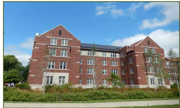
Rooftop Solar, CERTs
