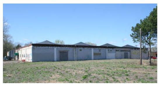
Figure 48. Northeast (side) and southeast (rear) elevations of the warehouse showing pyramidal roof structure, view facing northwest.
