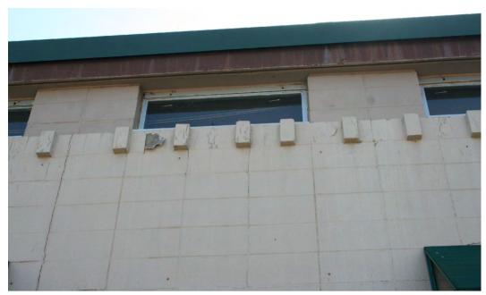
Figure 43. Detail of concrete dentil work that encircles the warehouse, view facing southeast.
