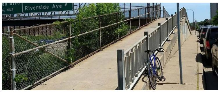
Figure 5 Non ADA compliant ramp system on South end
