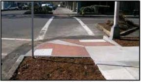
This curb ramp is an example of a design which could make it easier to fit two perpendicular curb ramps per comer than the current standard. Source: Accessible Public Rights of Way: Planning and Designing for Alterations, institute of Transportation Engineers, July 2007.
