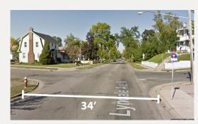
Typical existing cross section with an under-utilized parking lane, southbound travel lane, and northbound curbside travel lane.
