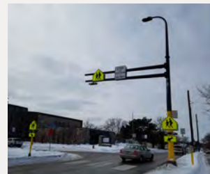
Traffic control device and APS push buttons
