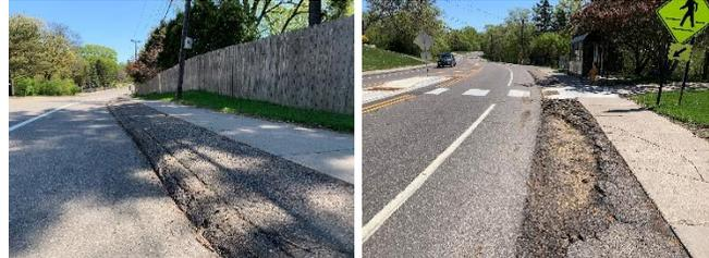
▲ **Golden Valley Road/ Bassett Creek Regional Trail alignment:** current conditions include multiple patched surface types that are failing/ heaving.
