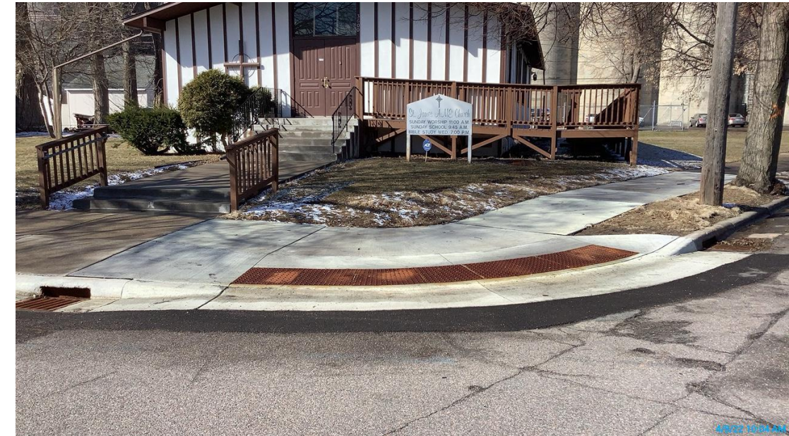
ADA improvements on local street corner – bringing substandard facilities up to ADA accessibility standards
