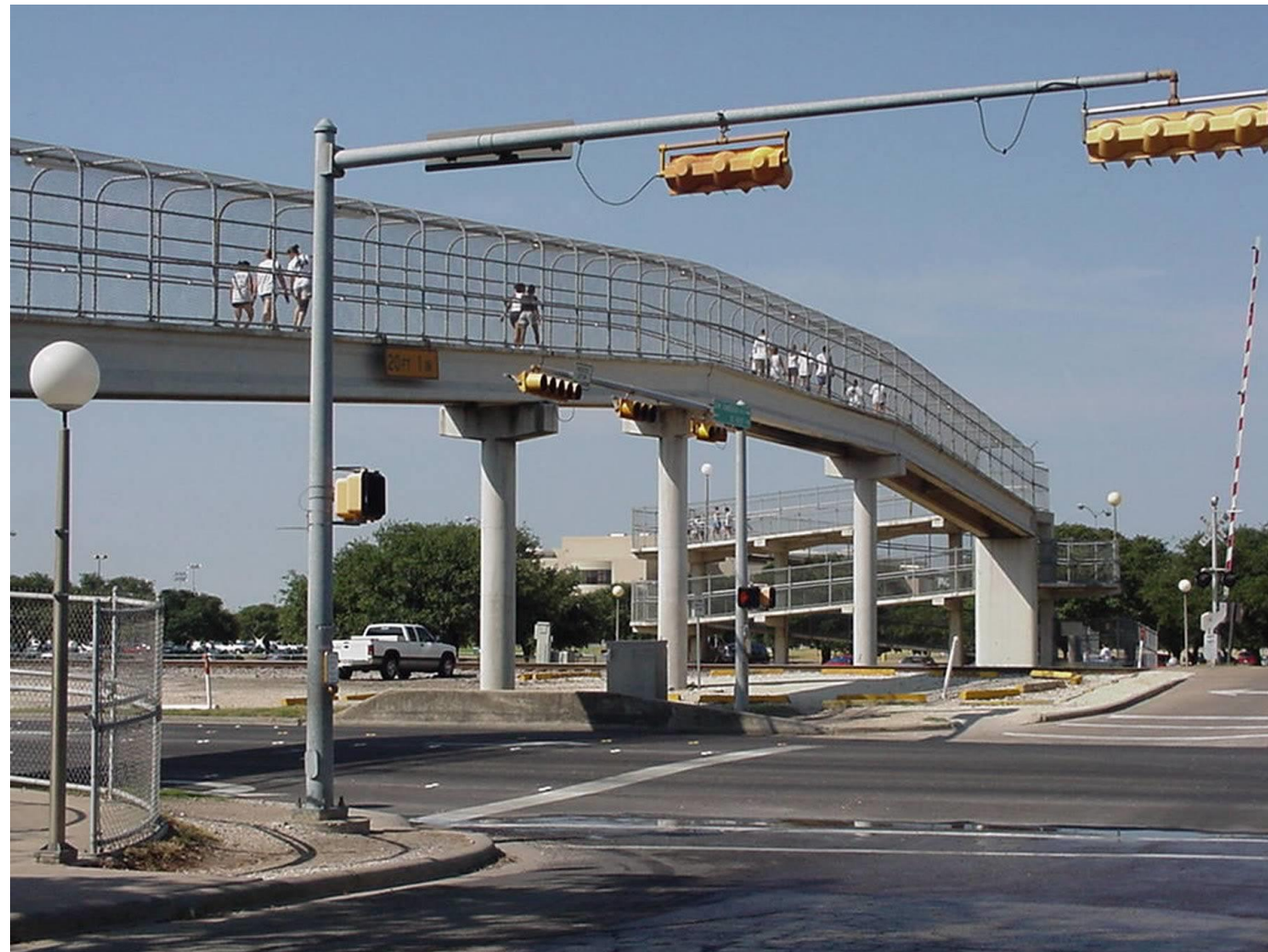
Ped/Bike Bridge - www.pedbikeimages.org - Dan Burden
