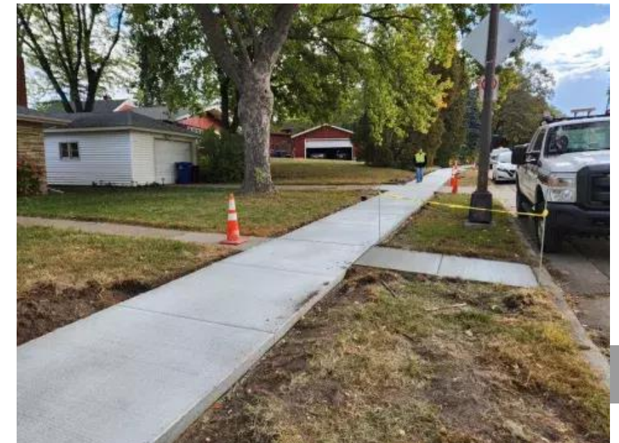
Typical St Paul concrete sidewalk – filling in sidewalk gaps
