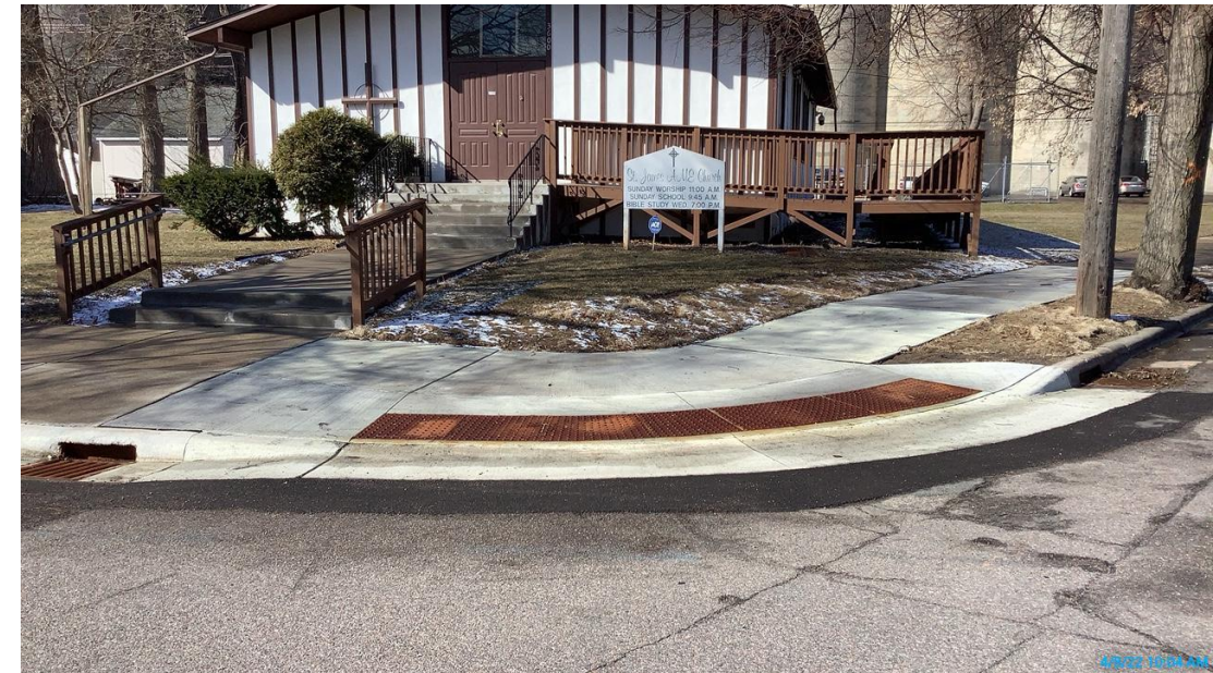
ADA improvements on local street corner
