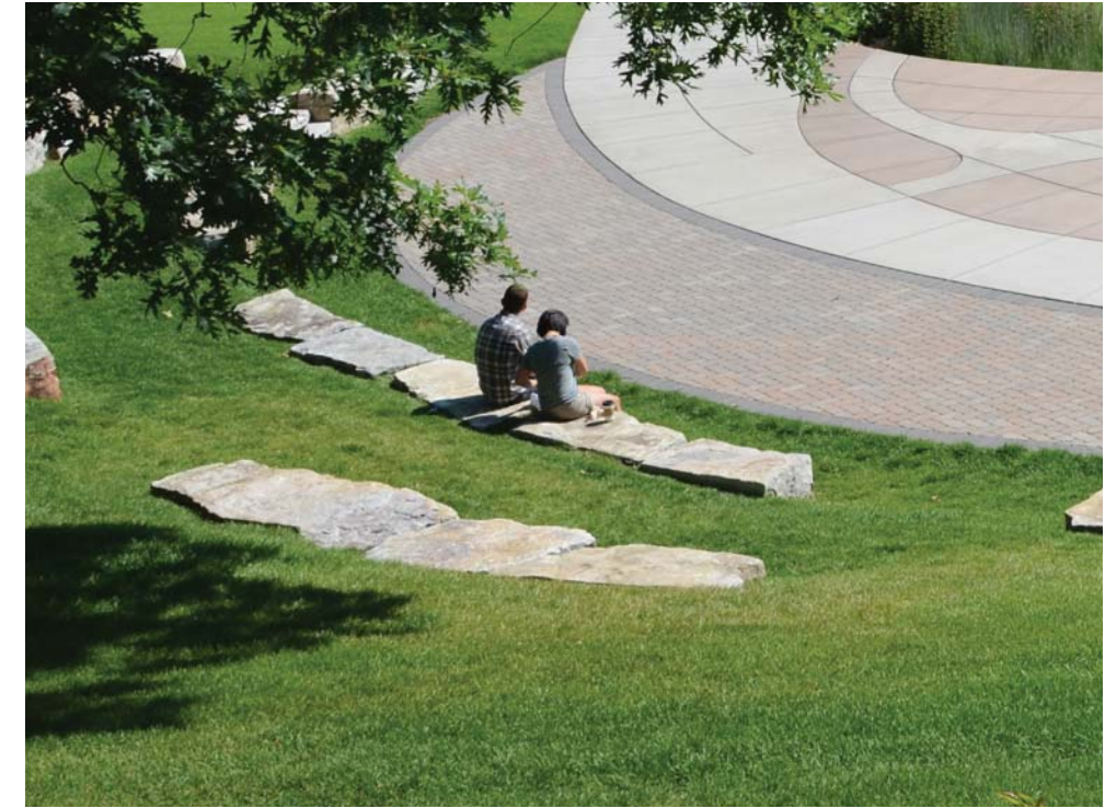
AMPHITHEATER LIMESTONE BLOCK SEATING
