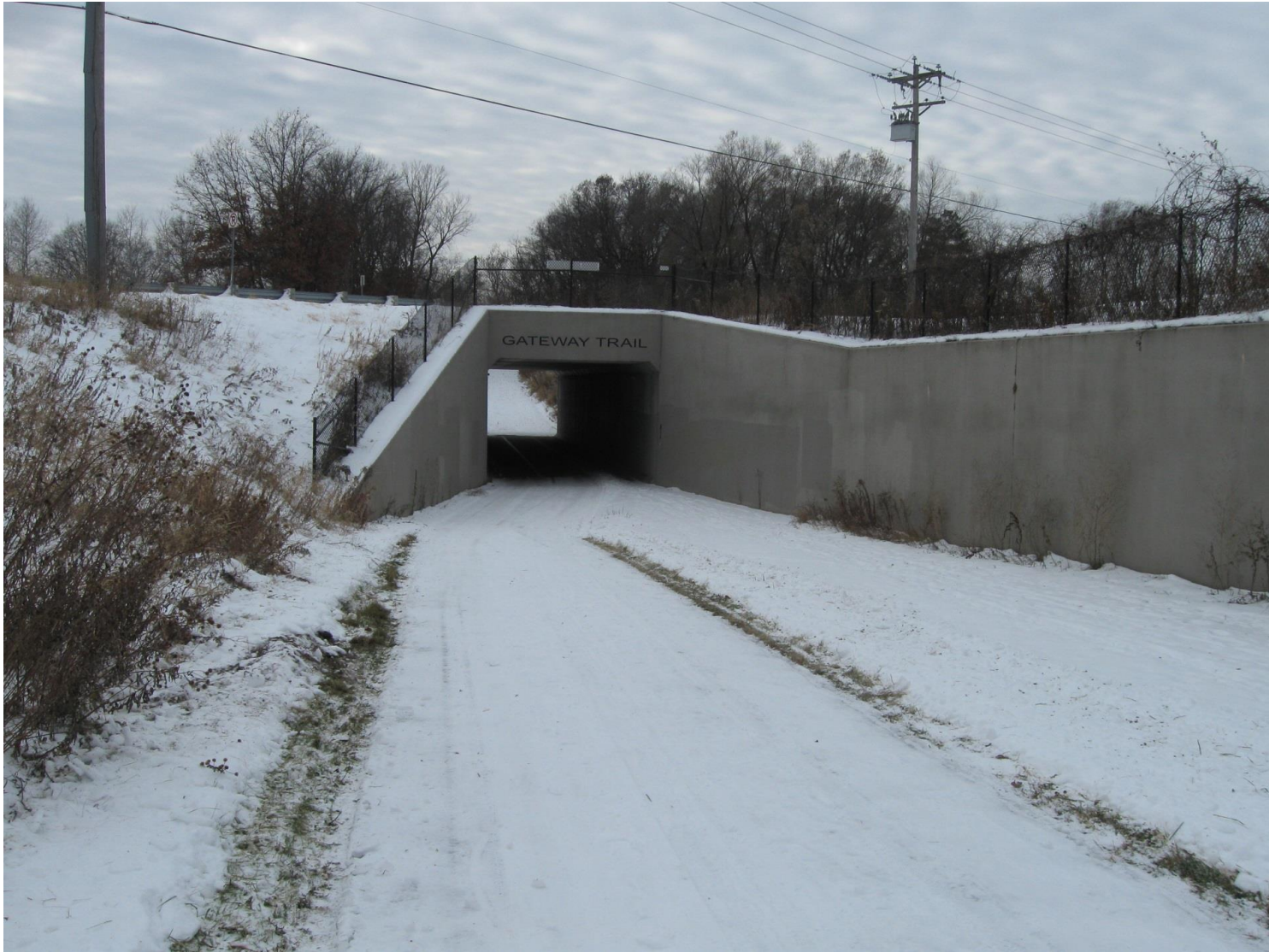
Example of Tunnel on Gateway State Trail at Highway 12
