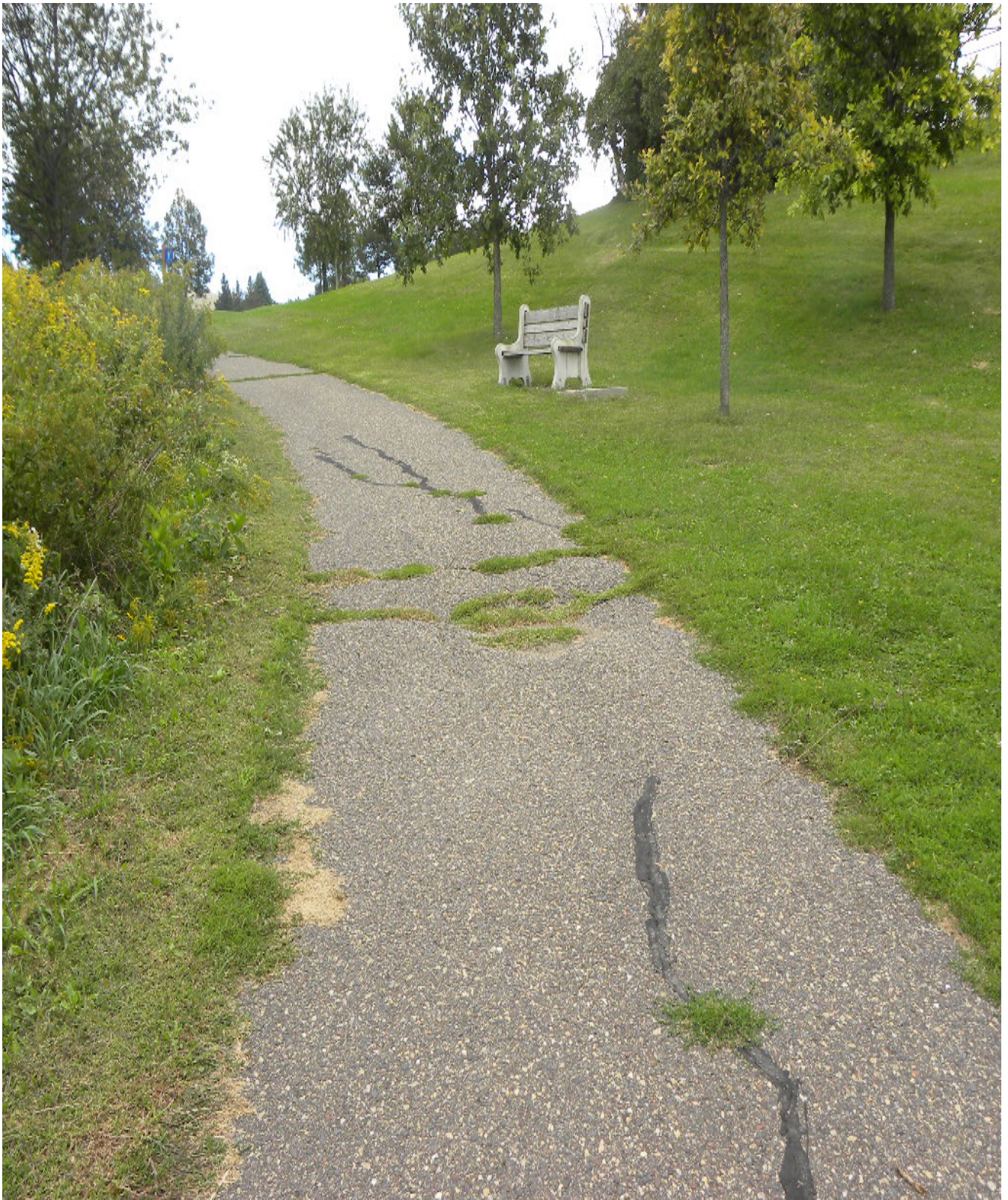
Existing trail conditions - 3
