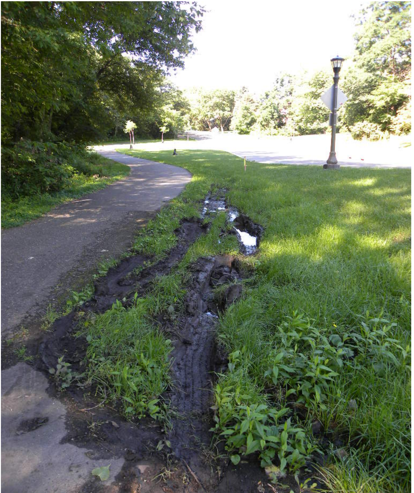
Existing trail conditions - 2
