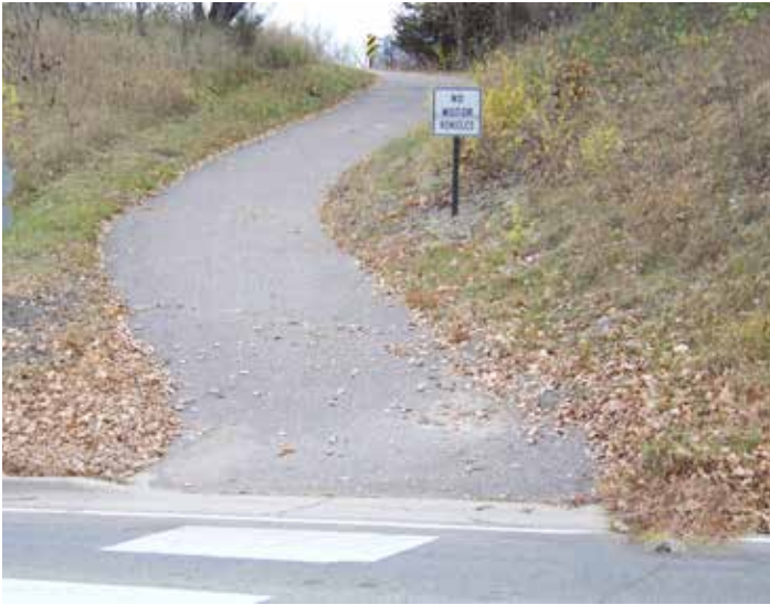
Looking west up at the western trail approach. The design of this approach forces trail users to navigate a 22 percent change in grade and then come to a complete stop at the roadway.
