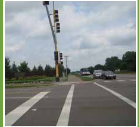
Intersection at Johnny Cake Ridge Road and 140th Street West
