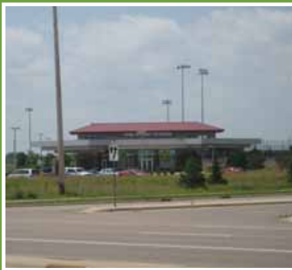
157th Street Transit Station
