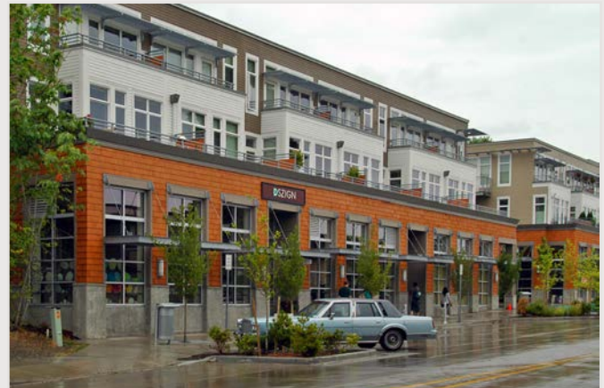
Mixed-use development with active street level uses
