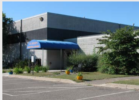
43 Hoops/County-owned development site
