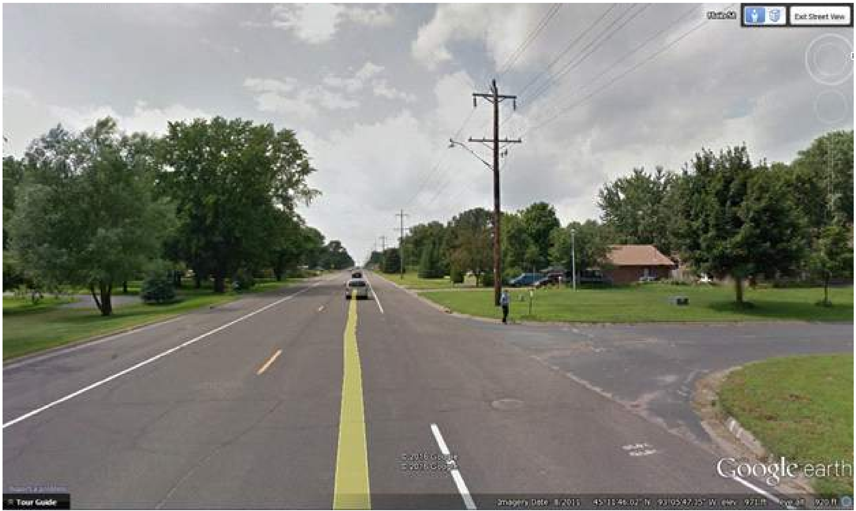
Figure 4b - CSAH 14 Urban Section at Elbe Street (looking west) Main Street (CSAH 14)/Central Anoka County Regional Trail Segment City of Lino Lakes Anoka County
